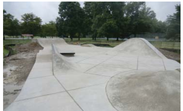
Handloff Park Skate Spot while still under construction.
