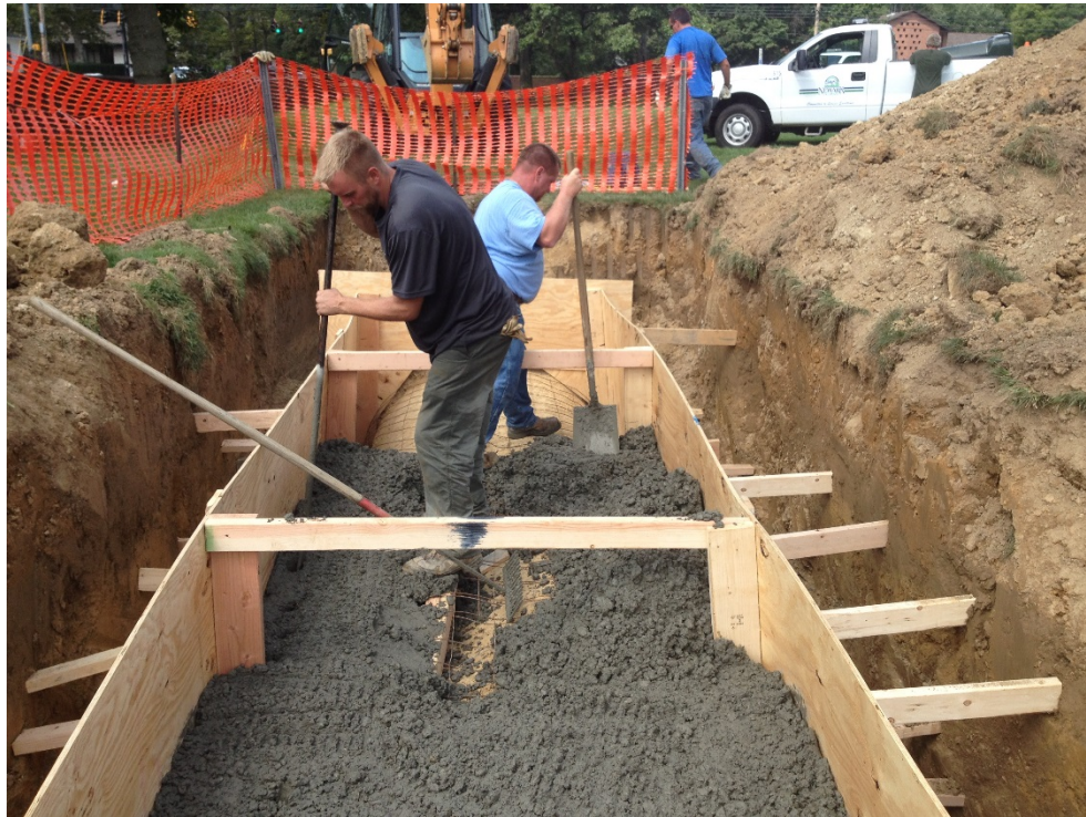
Figure 2: Concrete Support poured at Laurel Field
