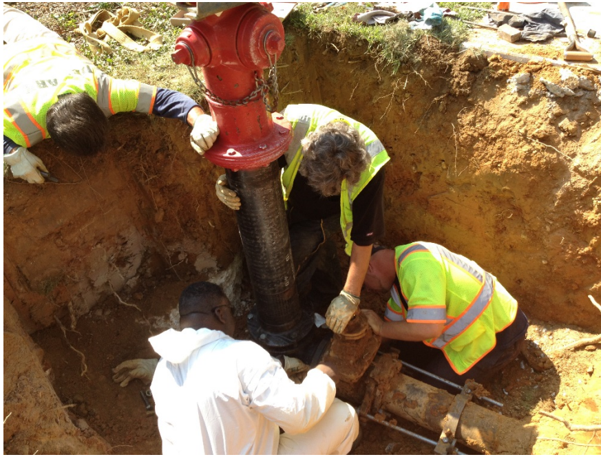
Figure 2: Fire Hydrant Replacement at Harvard Lane
