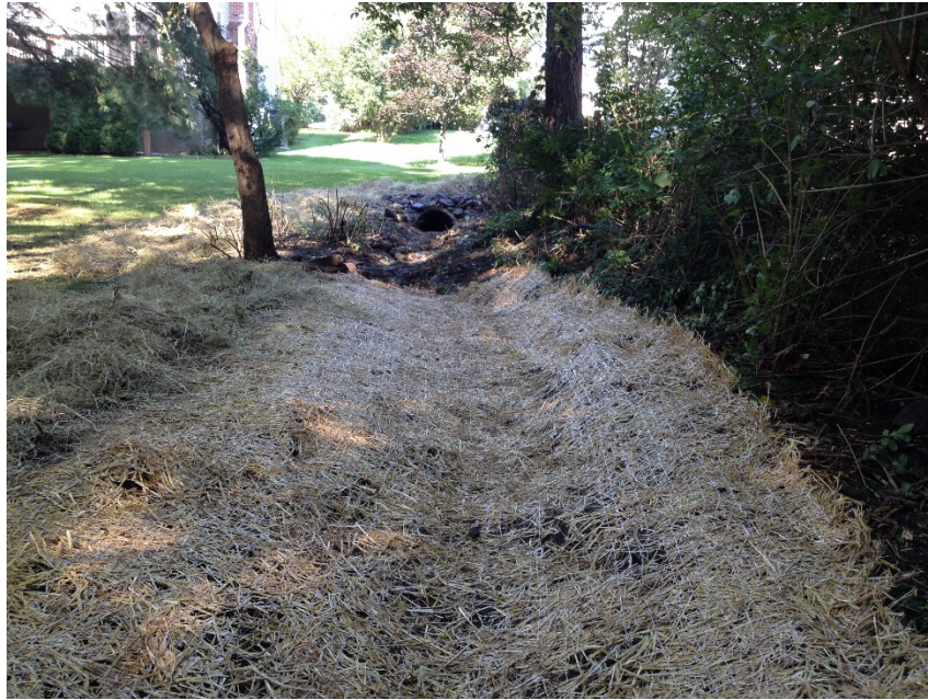
Figure 1: Storm Water Drainage Maintenance in Christianstead
