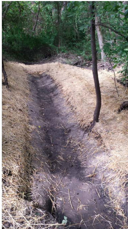
Figure 2: Storm Water Drainage Maintenance at Barksdale and Rahway
