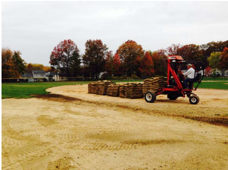
LeRoy Hill Park Drainage Project – Sod Application
