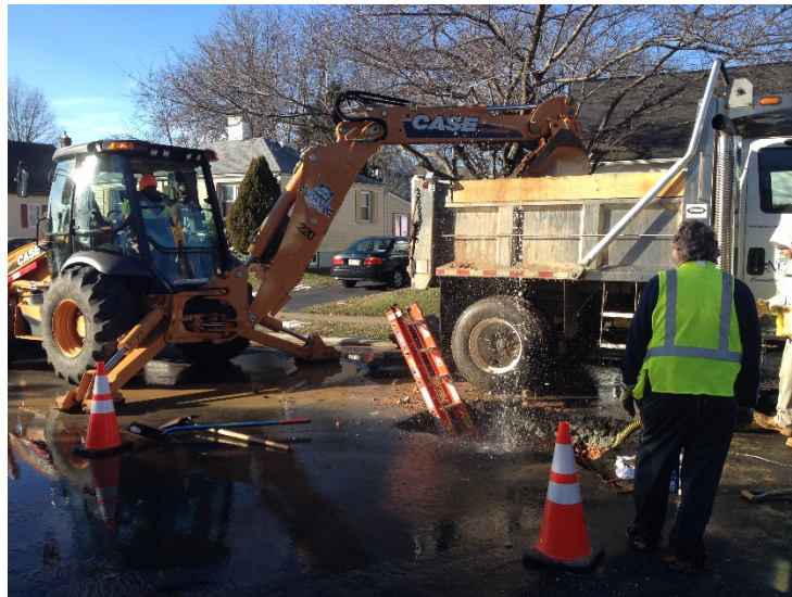
Water Main Break repair on 6" line at Tyre Avenue
