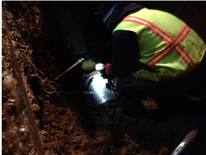
Water Main Break repair on 8" line at service connection on St. Regis Drive.
