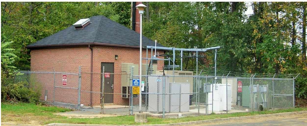
Figure 5: Example of a Core Site Facility
