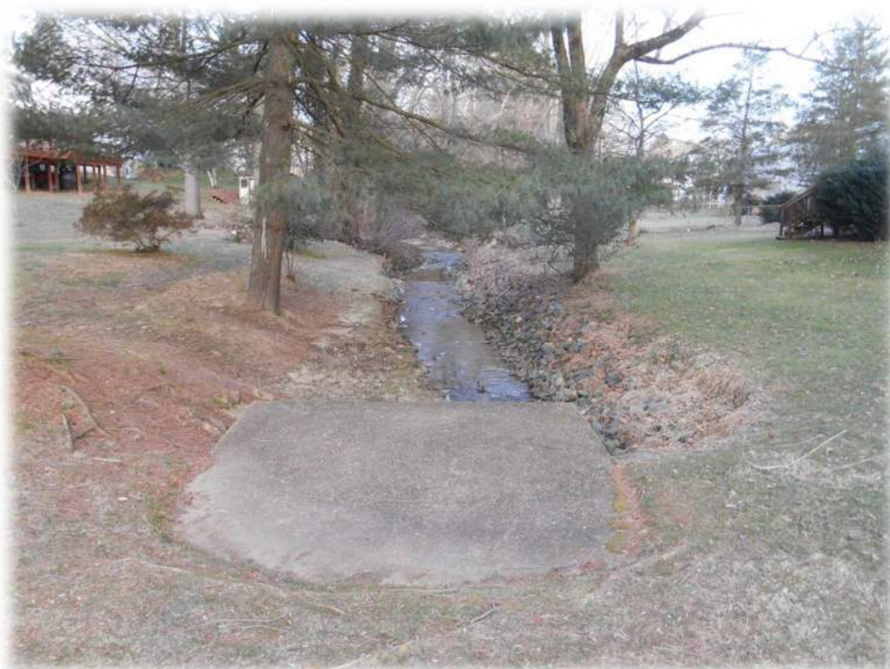
Figure 2 - Upstream Side of Box Culvert
