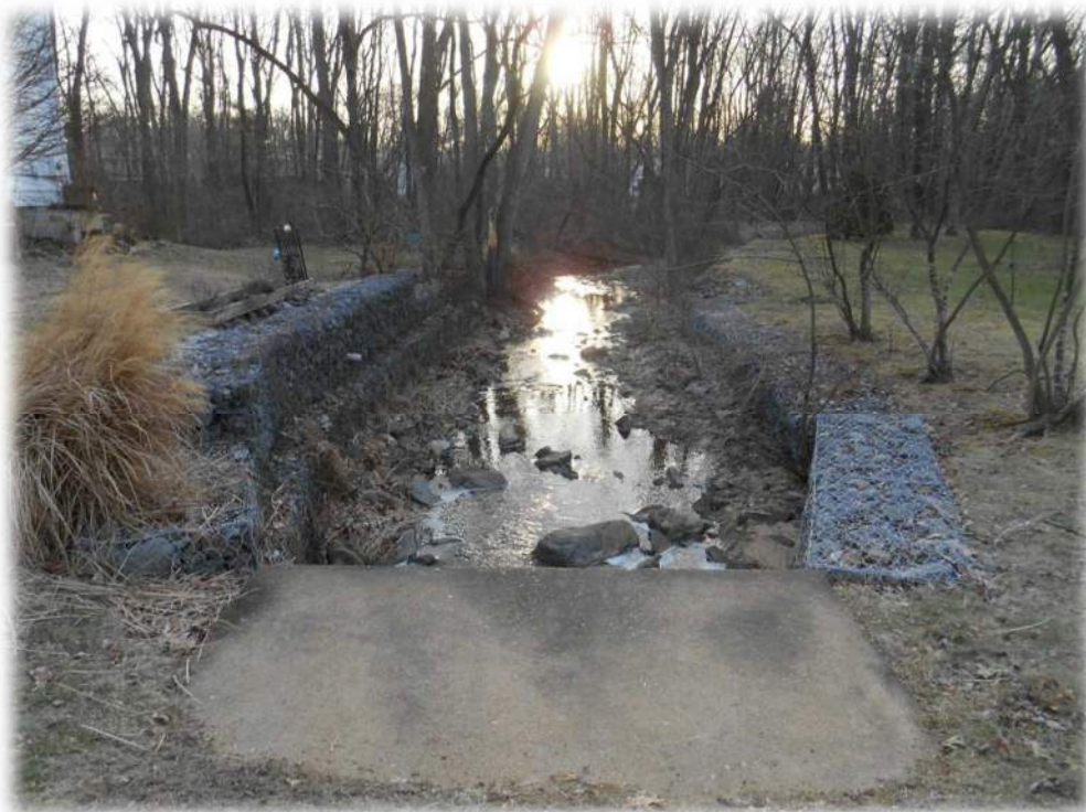
Figure 1 - Downstream Side of Box Culvert
