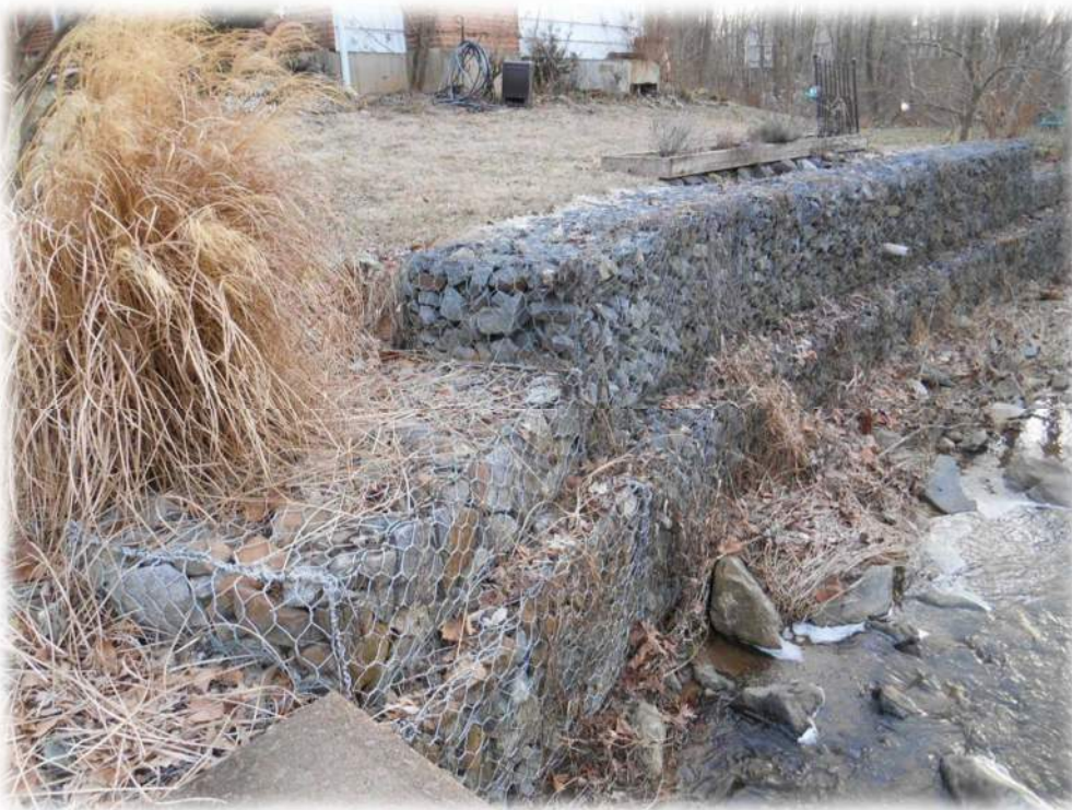
Figure 6 - Downstream Gabion Wall
