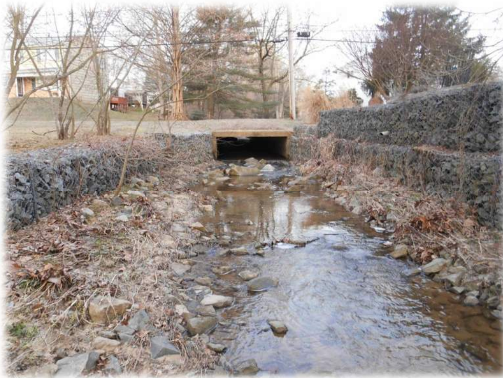
Figure 8 - Gabion Wall Channel Looking Upstream
