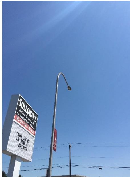
Figure 4.3.5 LED fixtures along Hwy 13.
