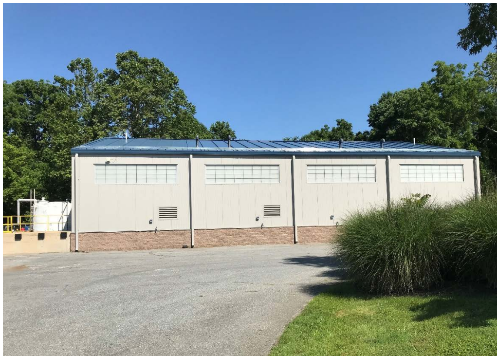
CITY OF NEWARK: CURTIS WATER TREATMENT PLANT
