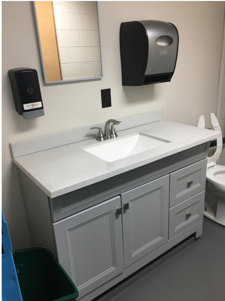
Rittenhouse bathroom remodel:
