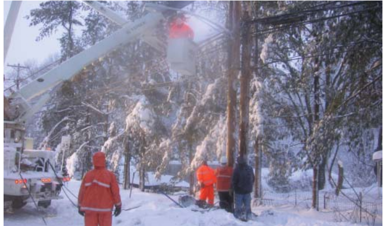
Newark Electric crews working through a snow storm to restore power
