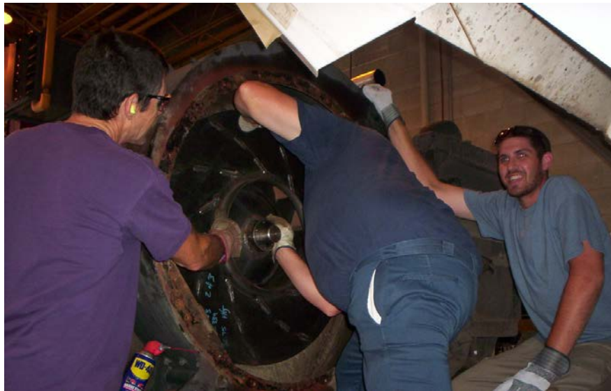
Figure 2: Sweeper Fan Replacement
