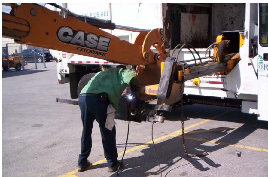
Figure 1: Side Loader Arm Welded Repair
