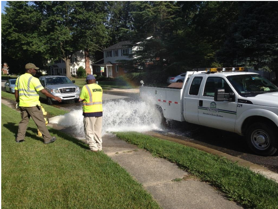
Figure 1: Water Main Flushing in Fairfield
