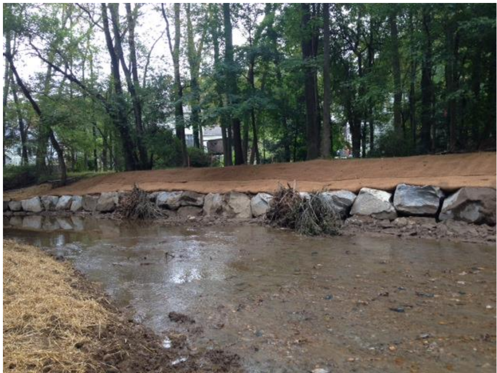
Rock wall with 2 root wads
