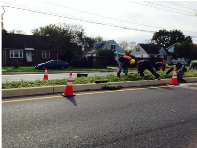
DeIDOT landscape contractor replacing plantings on Elkton Road.
