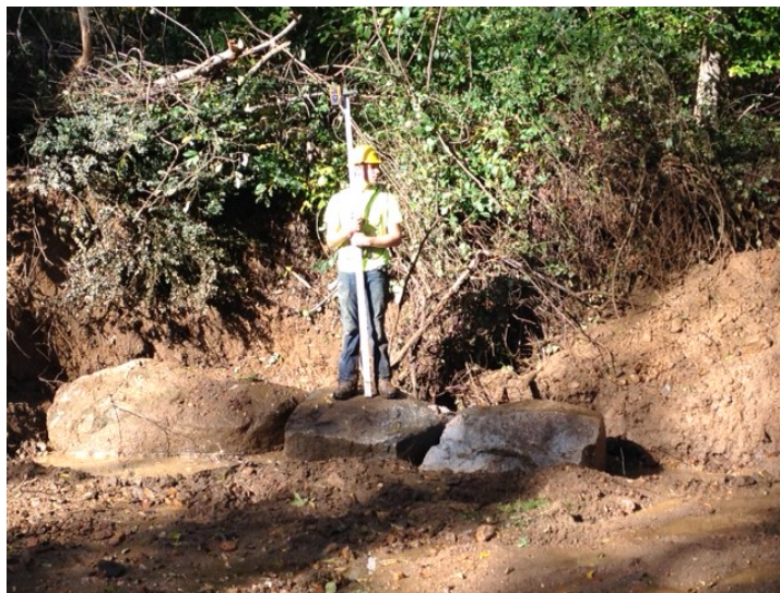
Checking grades during a rock vane installation
