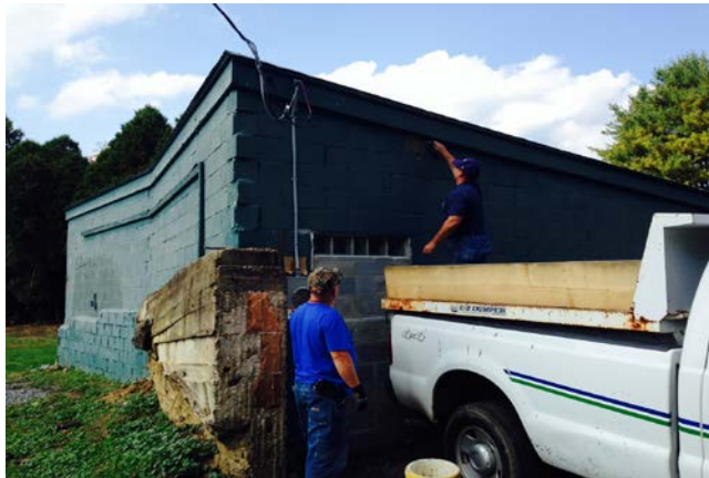
Parks crew members working on Community Garden building at Fairfield Park.
