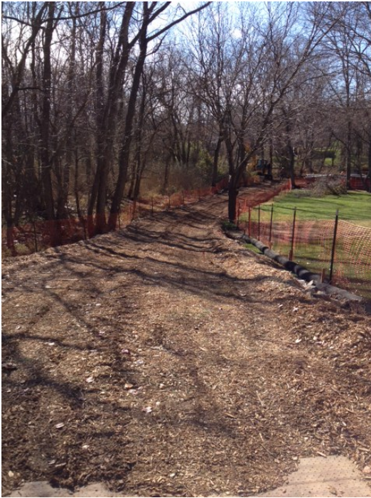
Phase II access road at Hidden Valley park.
