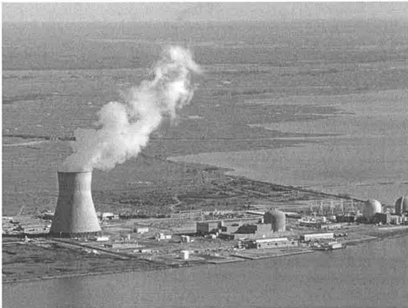
Artificial Island on the Delaware River in New Jersey is shown. Costs a transmission line project will be borne by Delaware, Maryland, Virginia and New Jersey residential, commercial and industrial consumers. (Photo: GARY EMEIGH/THE NEWS JOURNAL)
