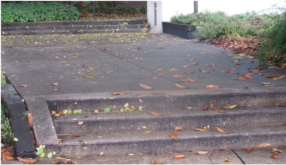
Images #13 and 14: Stairs to City Hall from South Main Street bus station.
