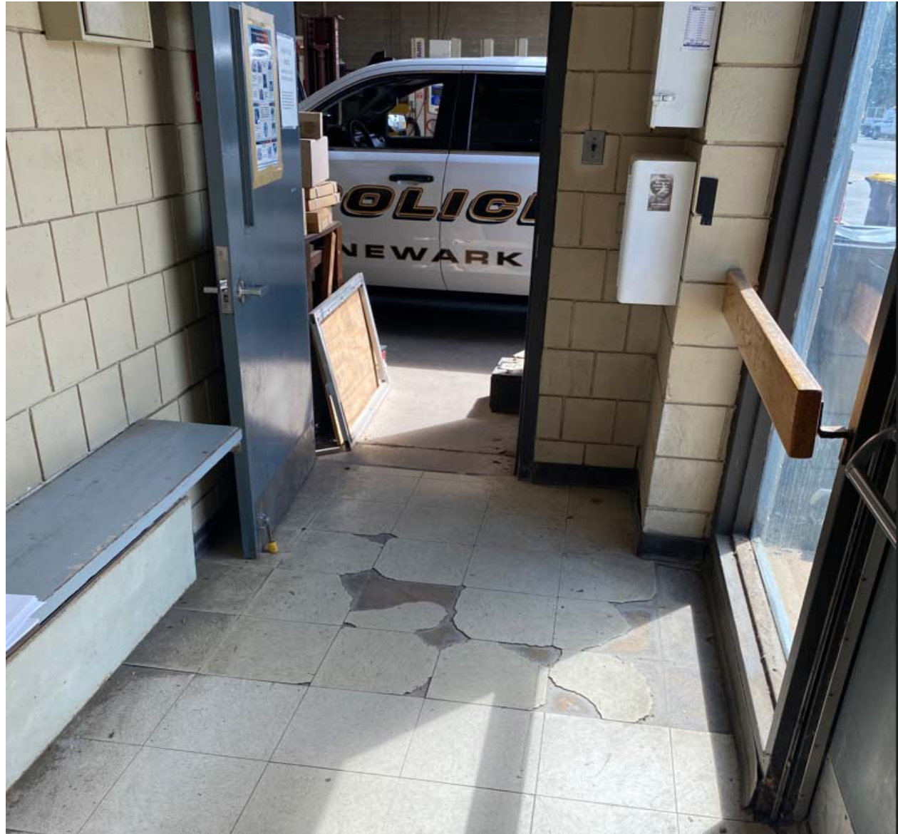
Image #1: FOC Building 1 (Electric and PWWR offices):
