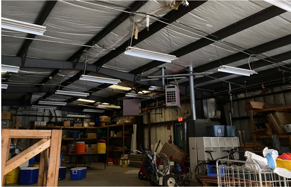
Images #19 and 20: FOC Building 4 (Parks Maintenance break room and offices):
