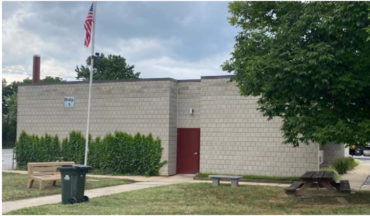
Images #11 and 12: FOC Building 1 (Electric and PWWR offices):
