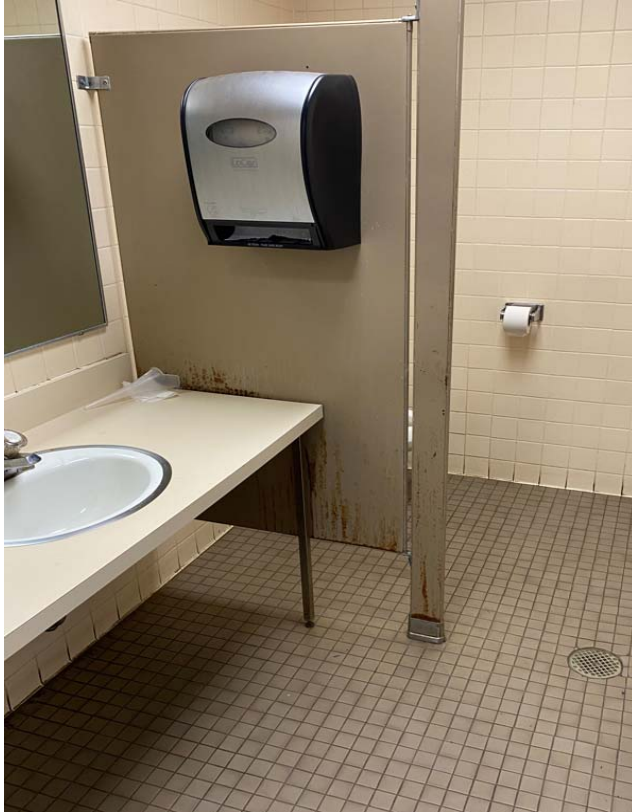
Images #21, 22 and 23: FOC Building 4 (Parks Maintenance break room and offices):
