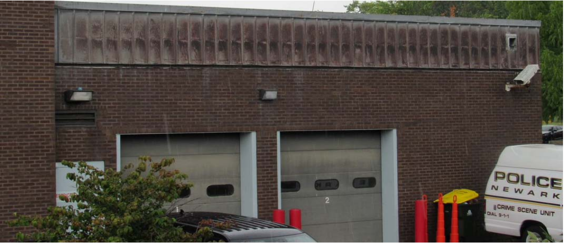
Images #21 and 22: Newark Police Department Sally Port (Apple Road view).
