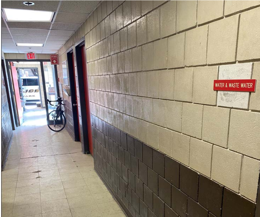
Images #9 and 10: FOC Building 1 (Electric and PWWR offices):
