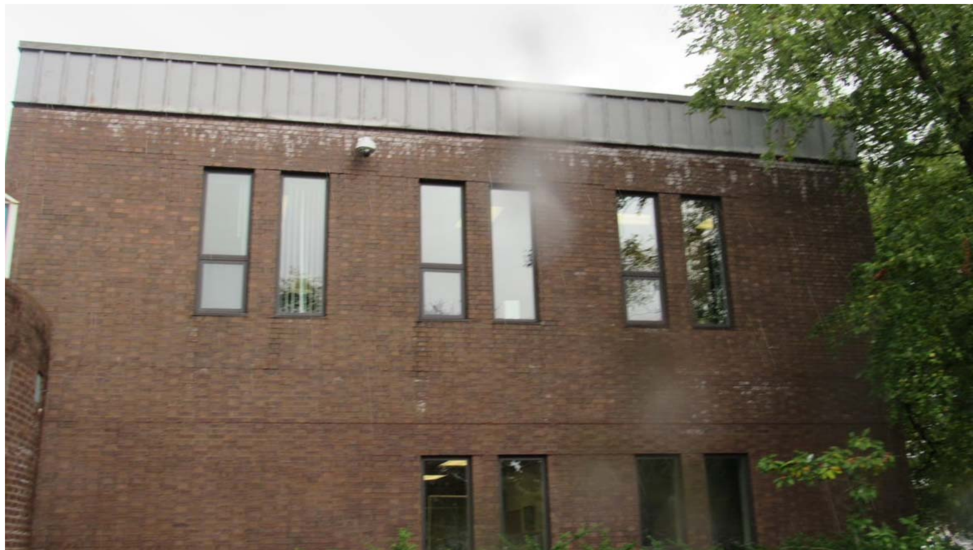
Image #29: City Manager's Office Exterior.
