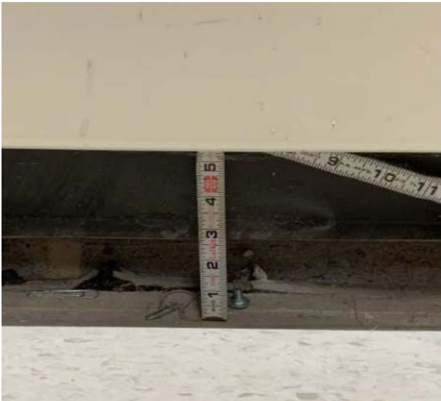
Images #1 and 2: Floor sinking and associated photographs
