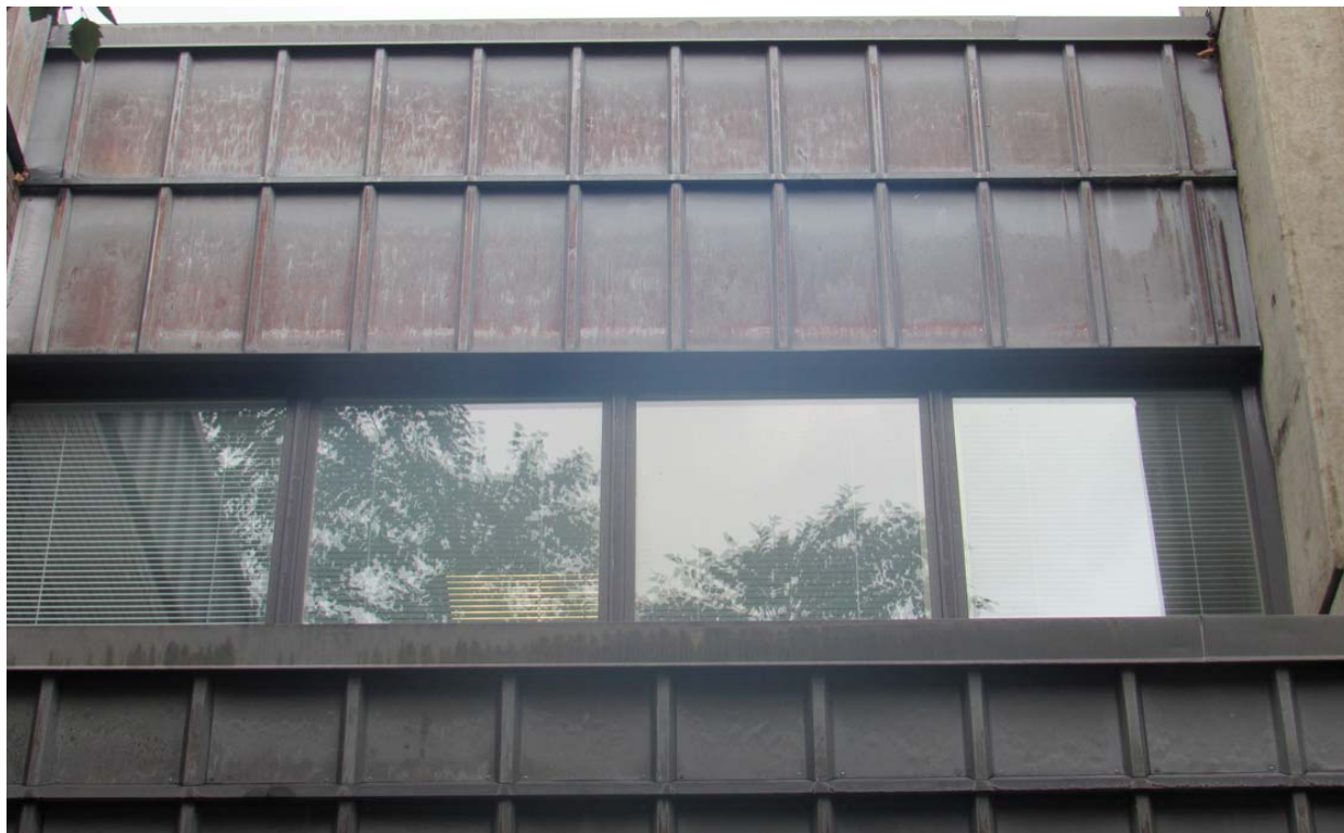
Images #7 and 8: South Main Street Side of City Hall.
