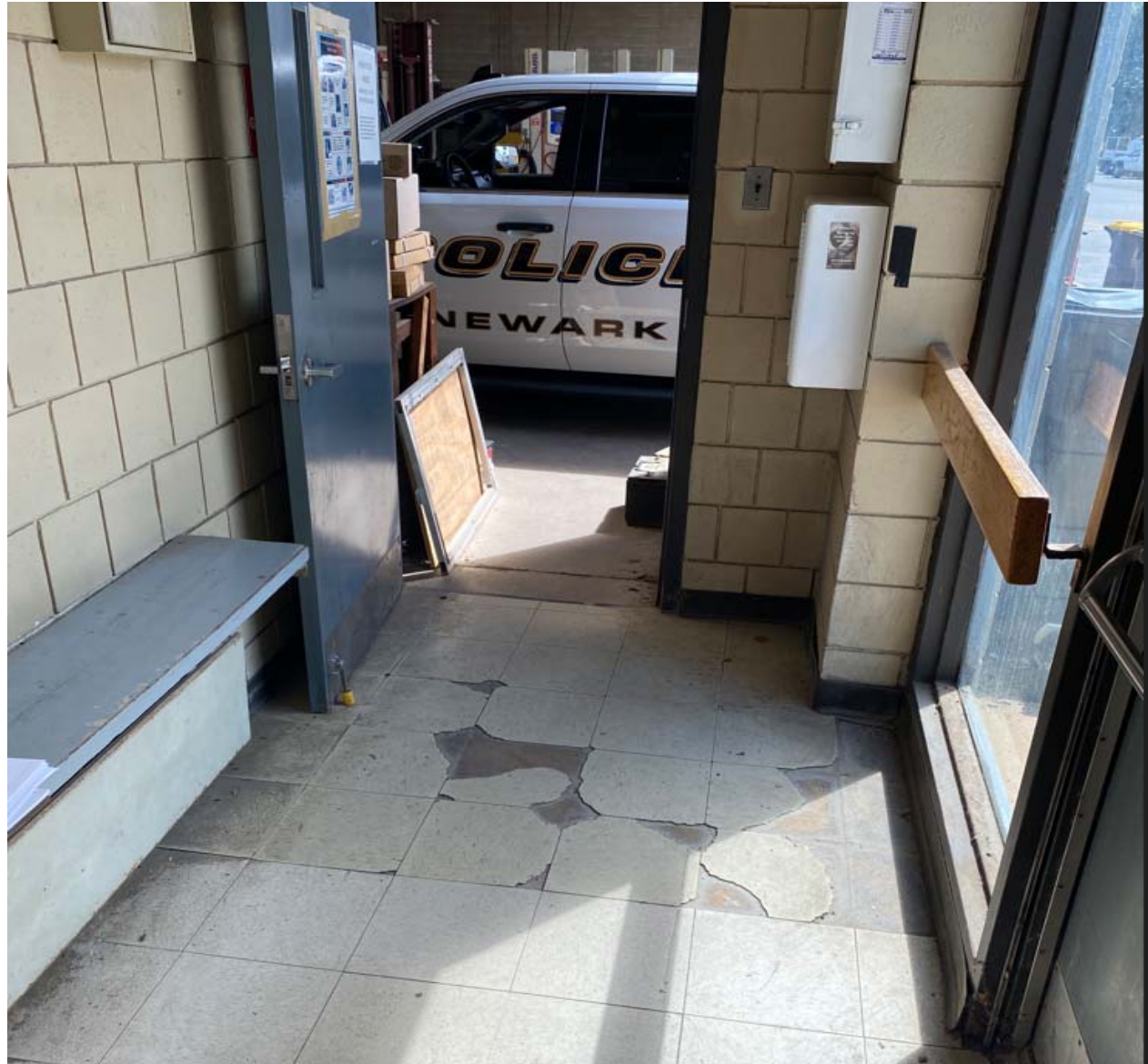
Image #1: FOC Building 1 (Electric and PWWR offices):
