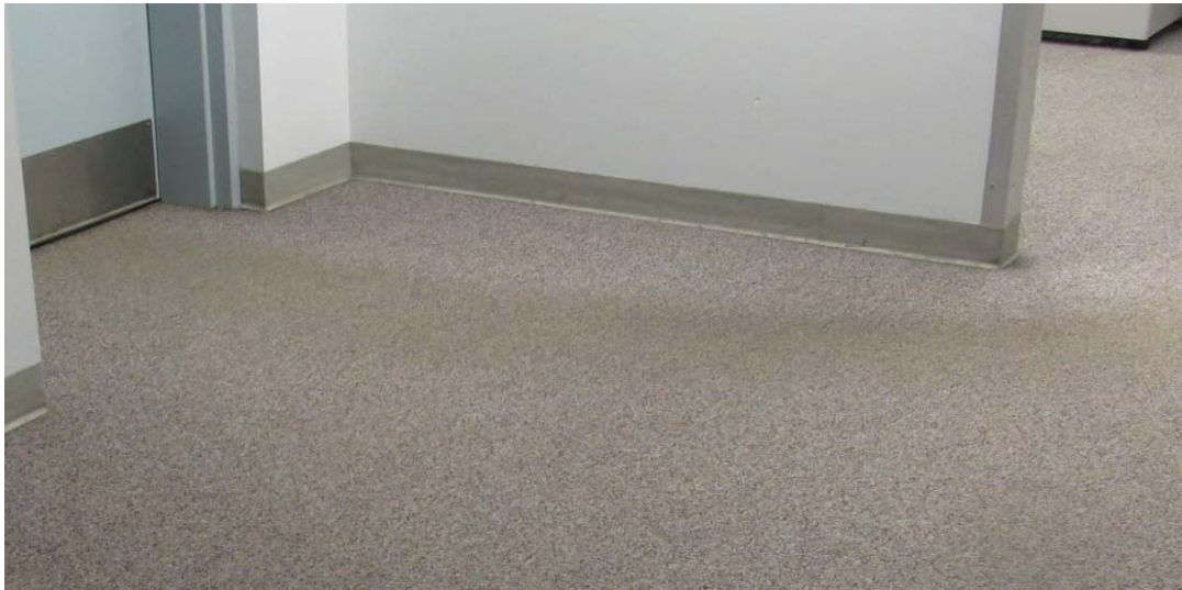
Images #6, 7 and 8: NPD 2nd floor hallway.
