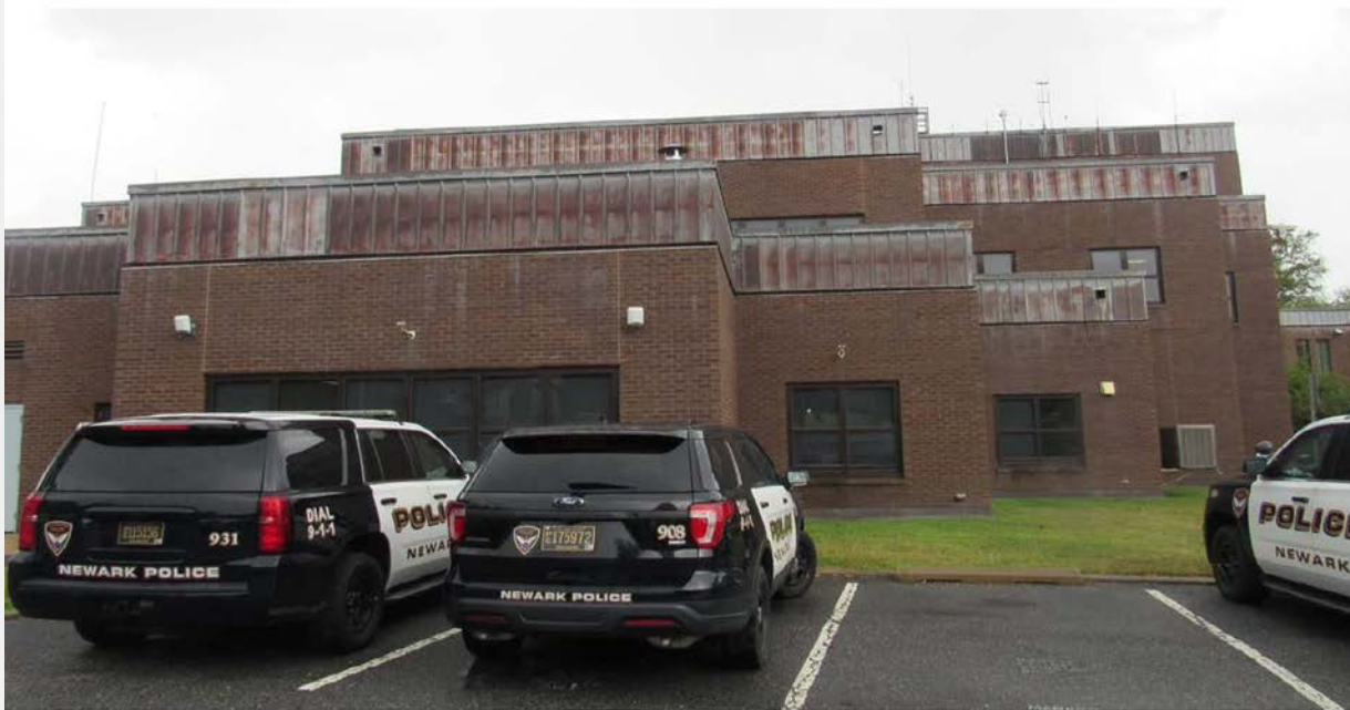
Image #18: Newark Police Department Sally Port (lot side).
