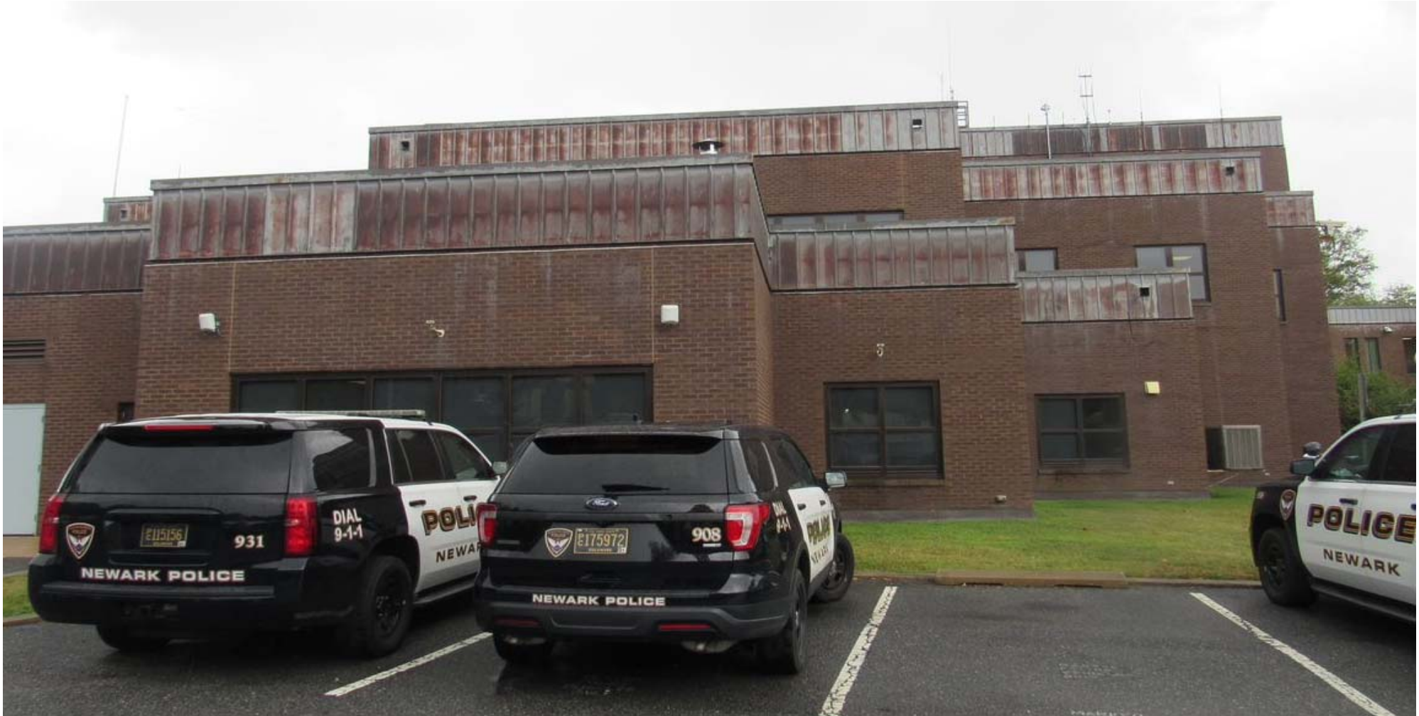
Image #24: Newark Police Department Sally Port (lot side).
