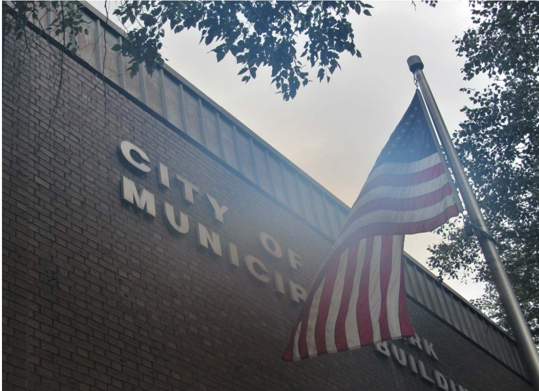
Images #9 and 10: South Main Street Side of City Hall.
