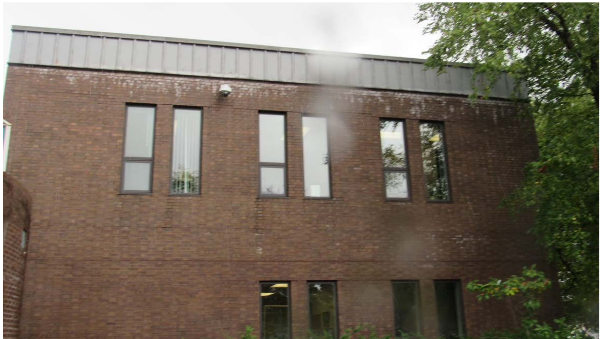
Image #29: City Manager's Office Exterior.
