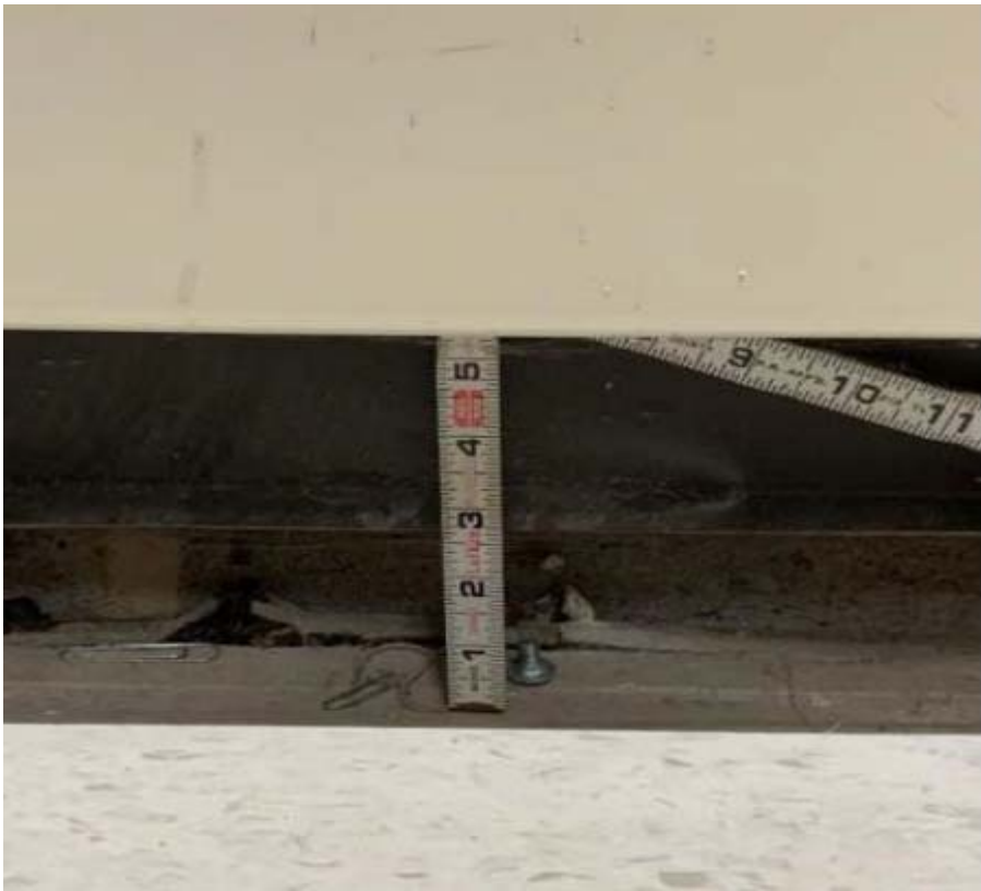
Images #1 and 2: Floor sinking and associated photographs
