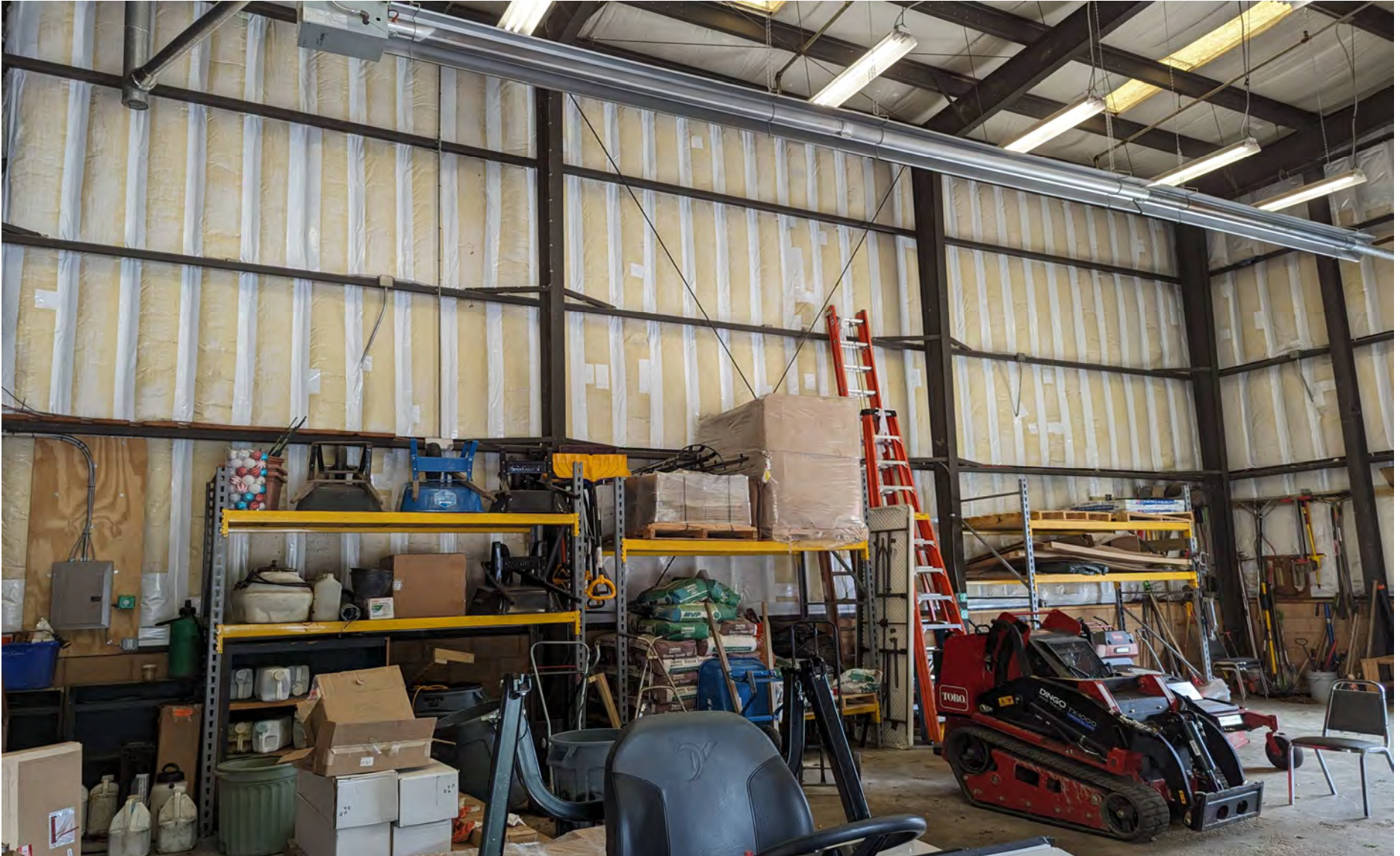
Image #14: FOC Building 4 - Repaired Insulation (AFTER).
