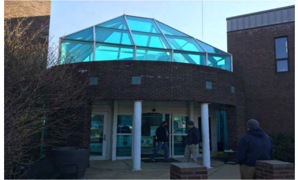
Image #2: Atrium Entrance (BEFORE).
