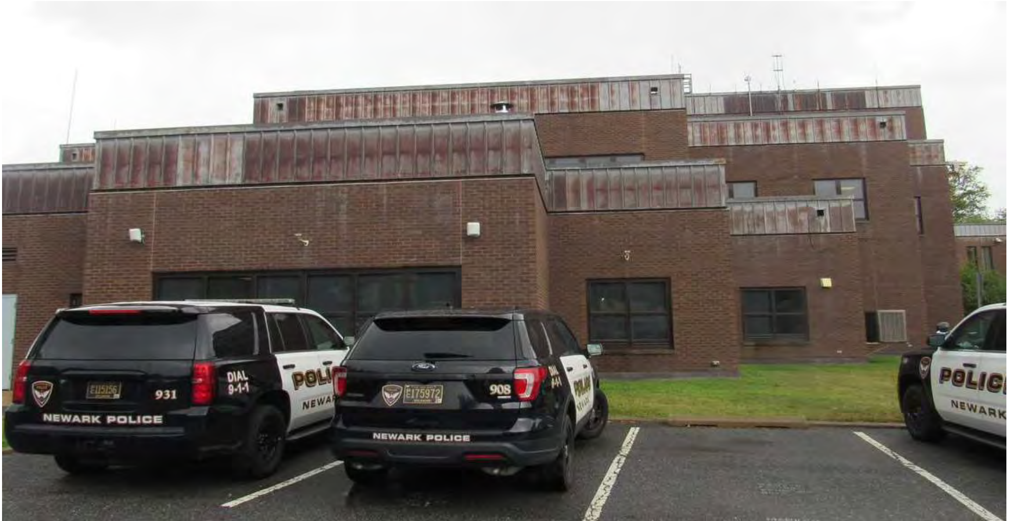
Image #25: Newark Police Department Sally Port (lot side).
