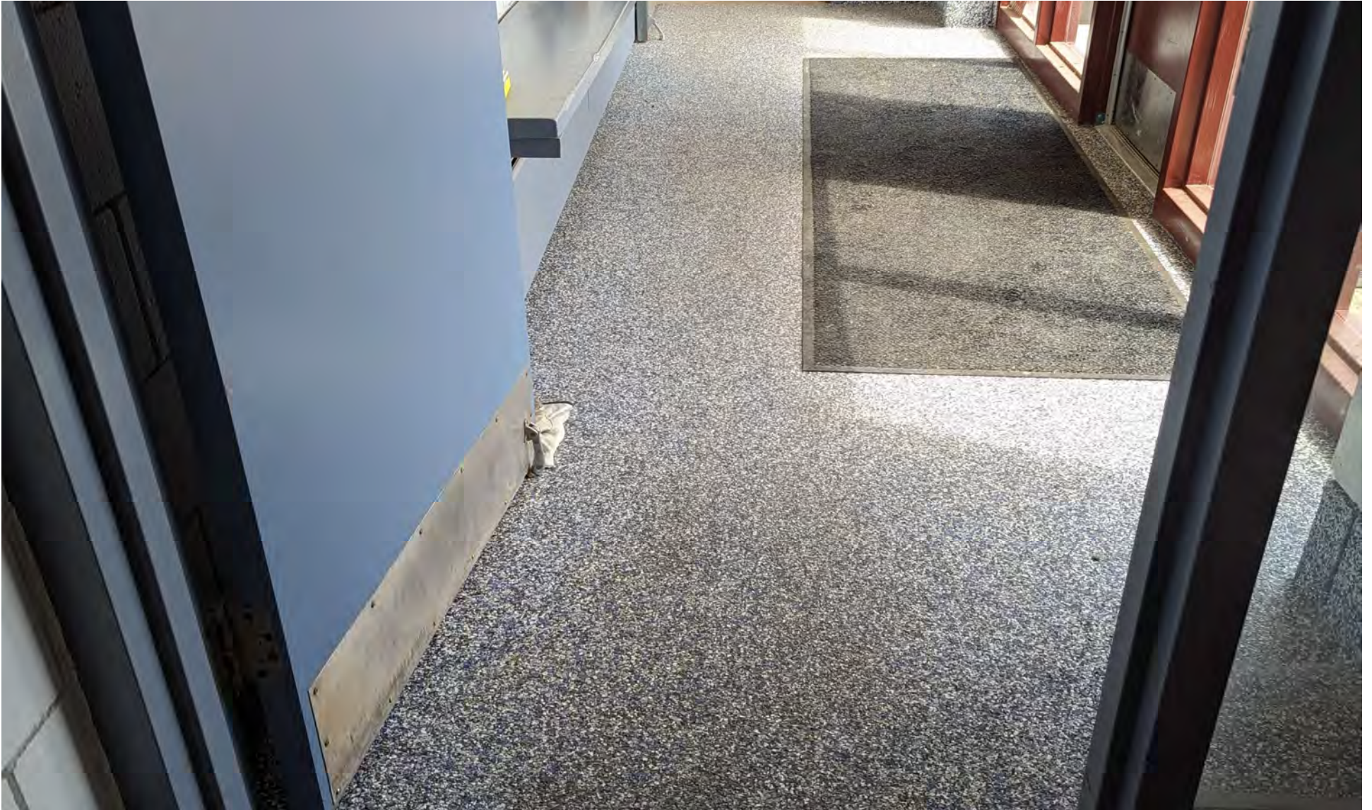
Image #6: FOC Building 1 - Repaired Flooring (AFTER).
