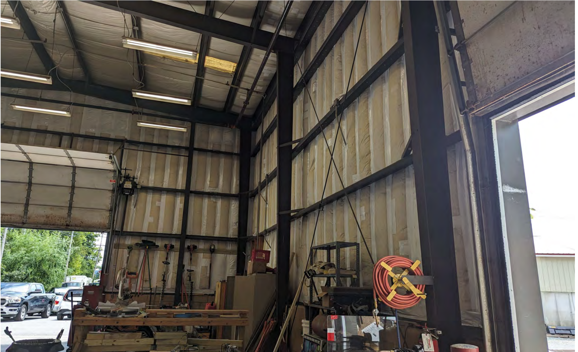
Image #13: FOC Building 4 - Repaired Insulation (AFTER).
