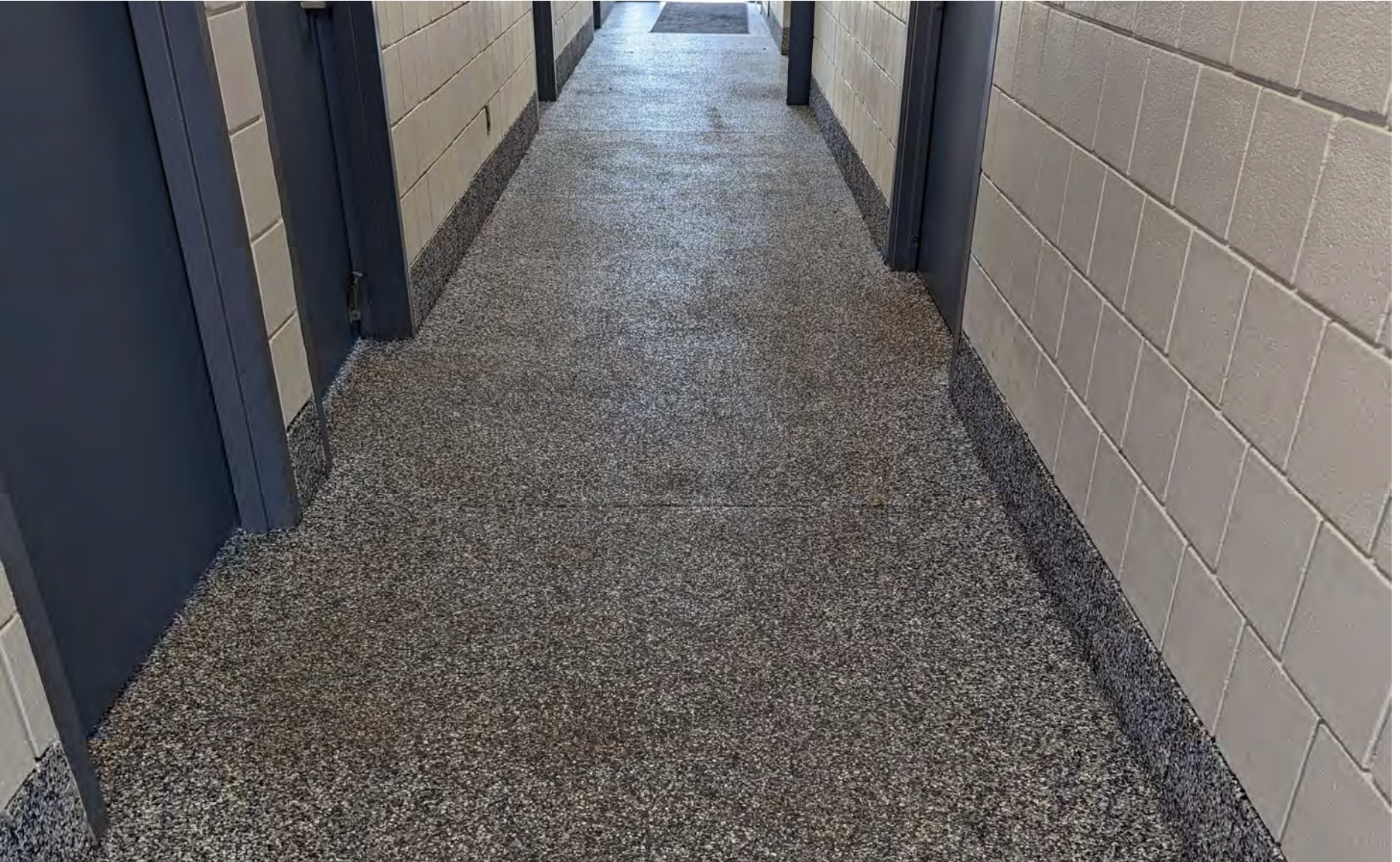
Image #5: FOC Building 1 - Repaired Flooring (AFTER).
