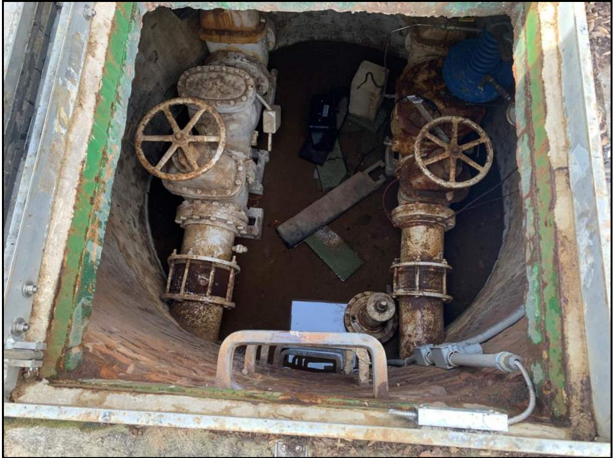
Arbour Park Valve Vault: Interior View of Valve Vault
