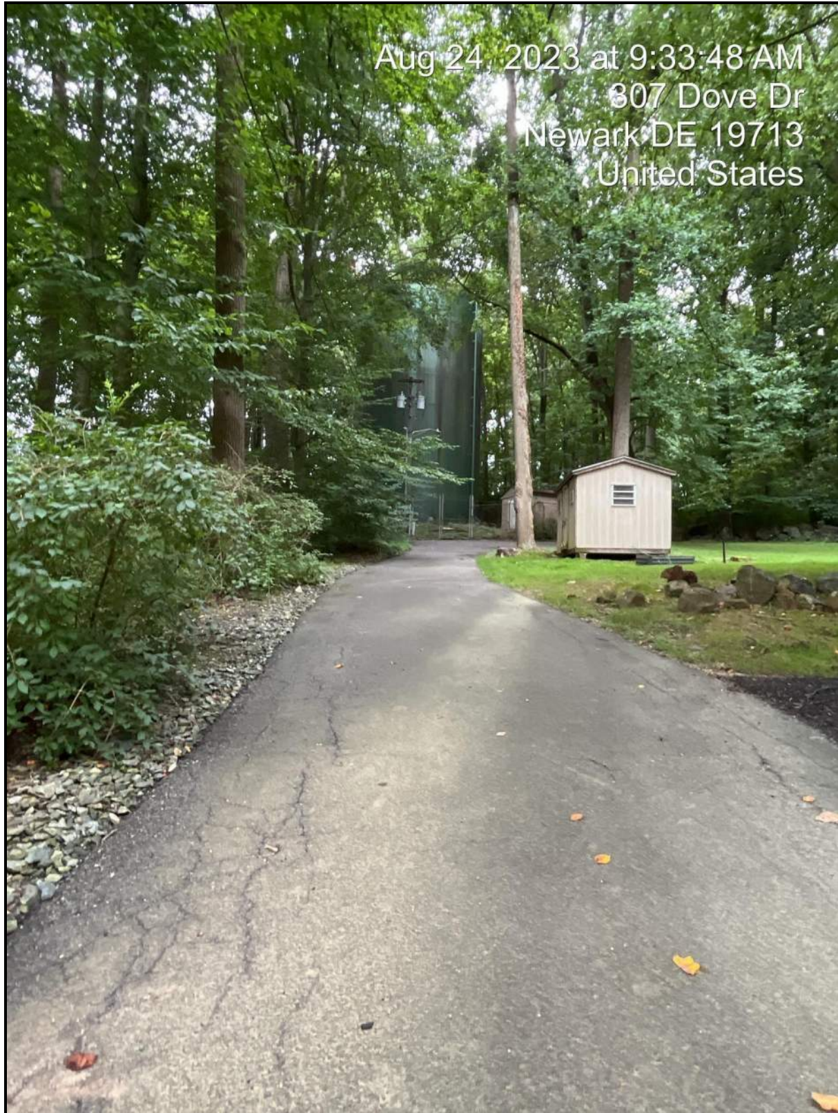
Arbour Park Valve Vault: Looking from Driveway to Vault Site
