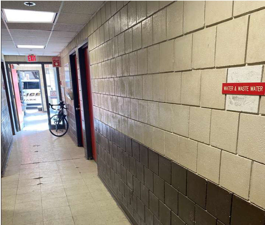
Images #3 and 4: FOC Building 1 [Electric and PWWR offices] (BEFORE).
