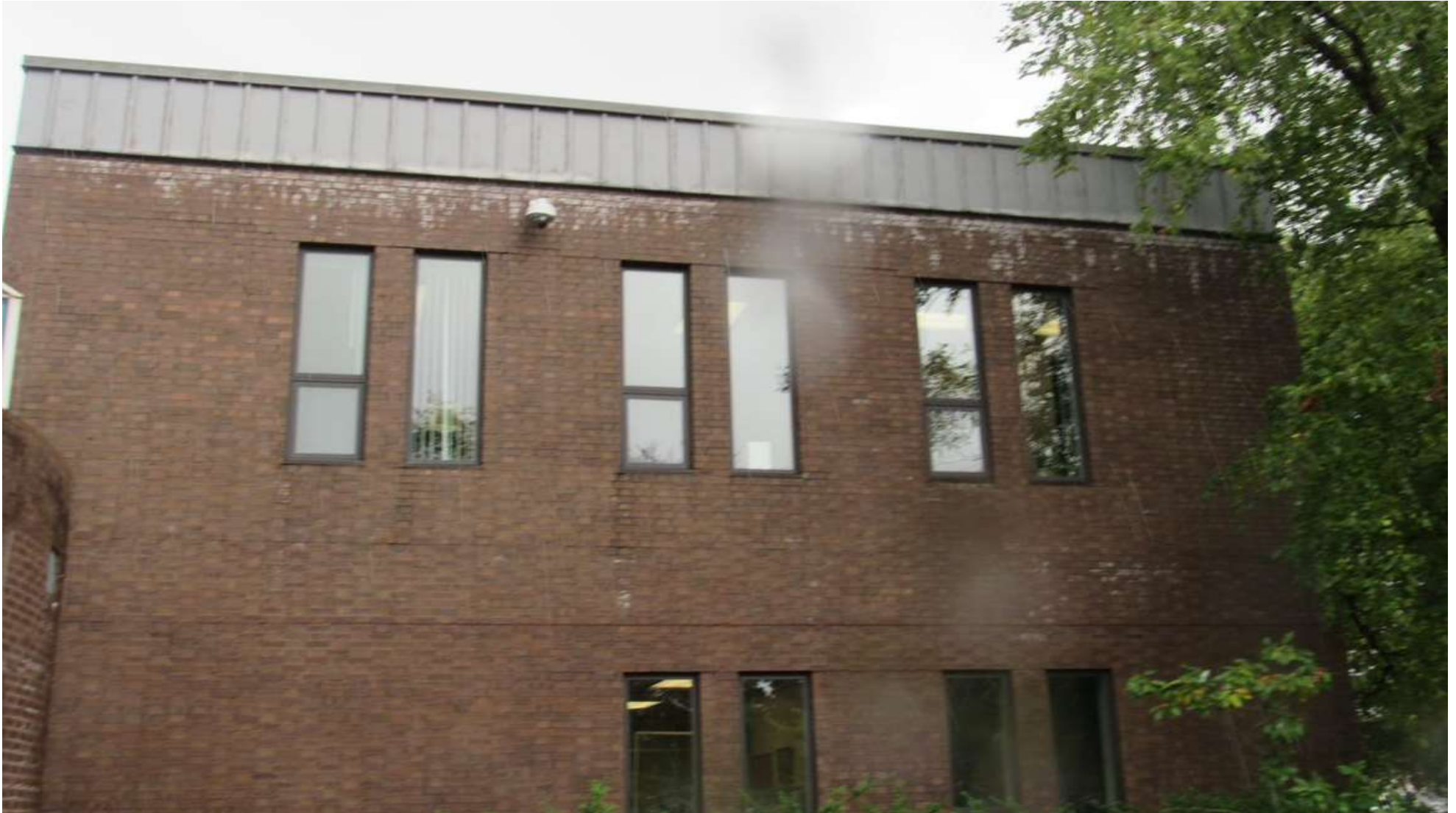
Image #30: City Manager's Office Exterior.
