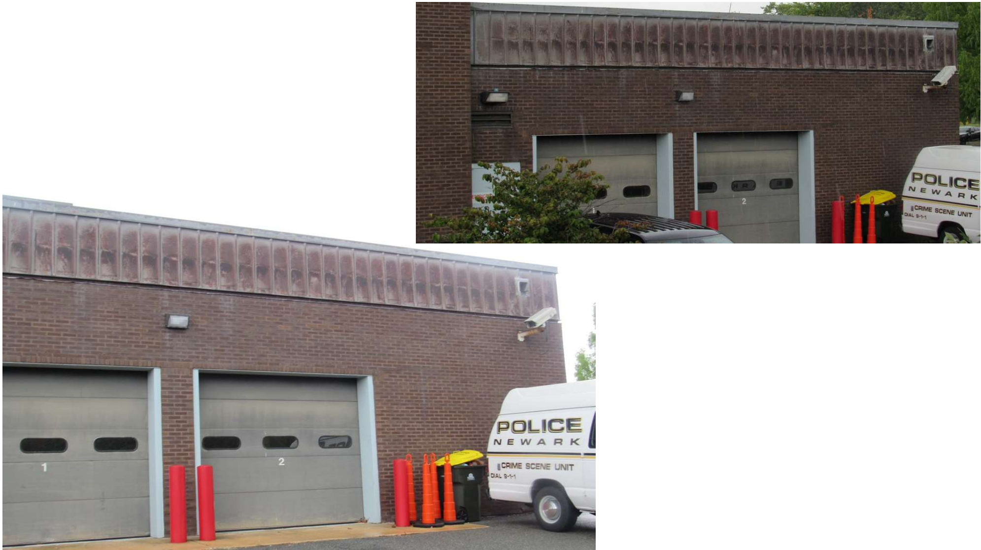
Images #22 and 23: Newark Police Department Sally Port (Apple Road view).
