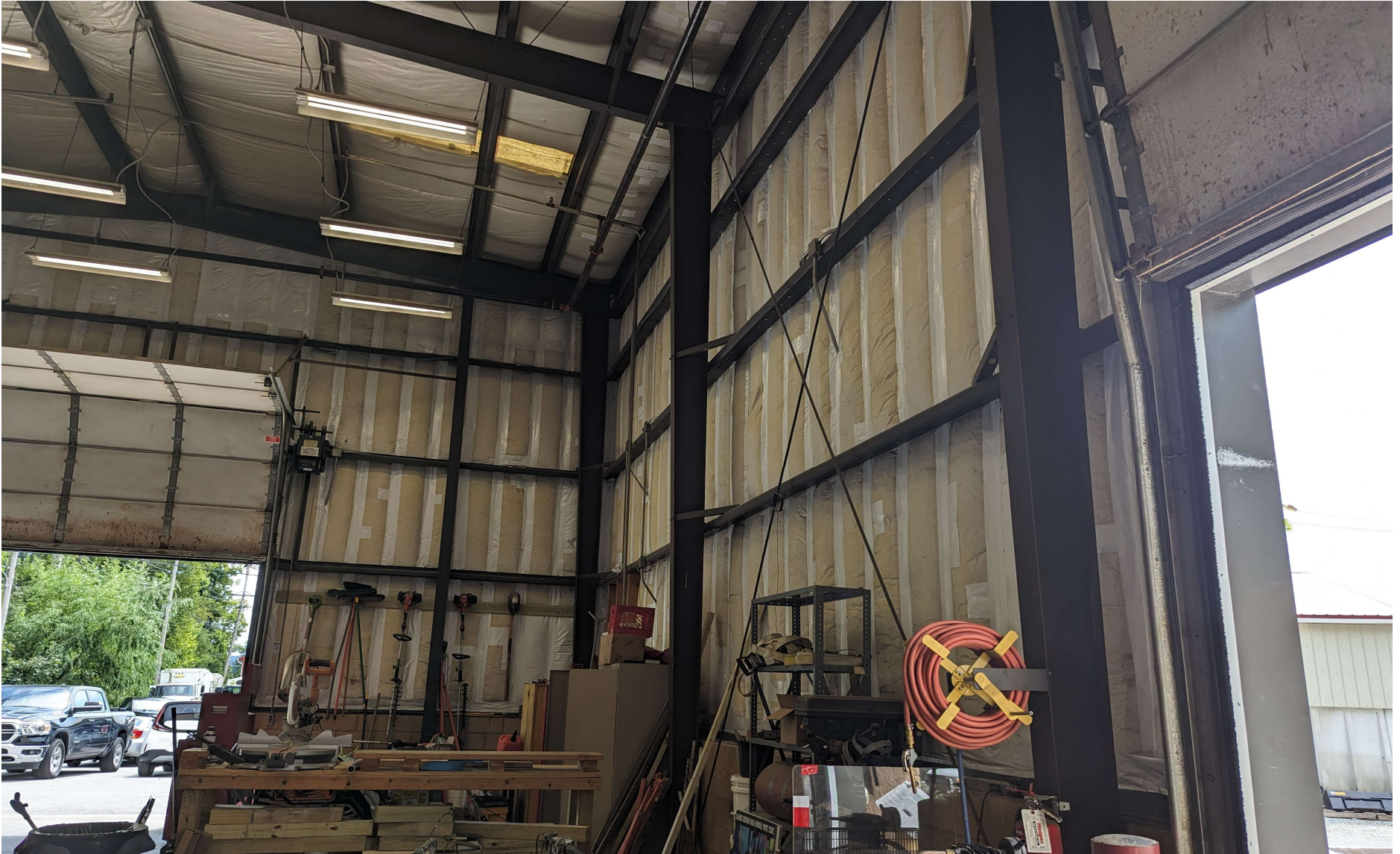
Image #13: FOC Building 4 - Repaired Insulation (AFTER).
