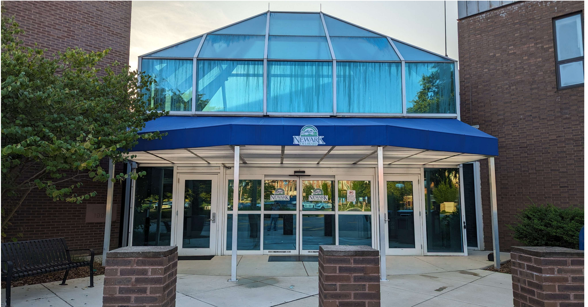
Image #5: Atrium Entrance (AFTER).
