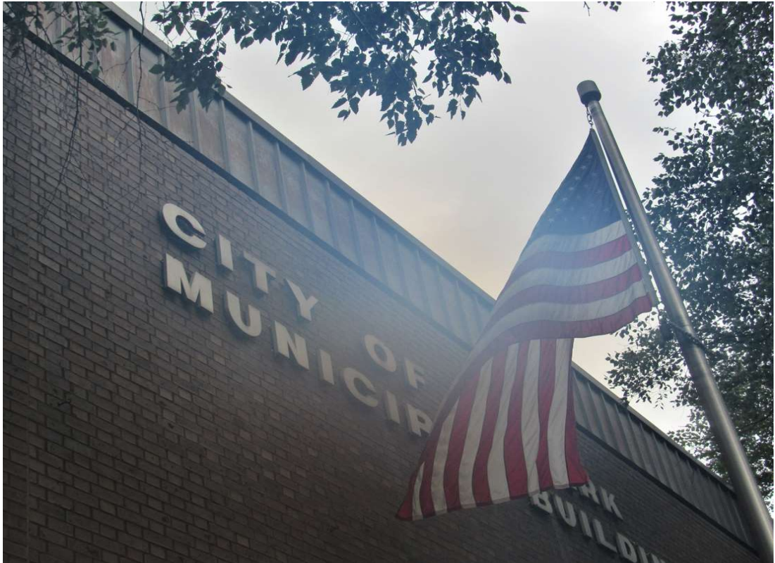
Images #10 and 11: South Main Street Side of City Hall.
