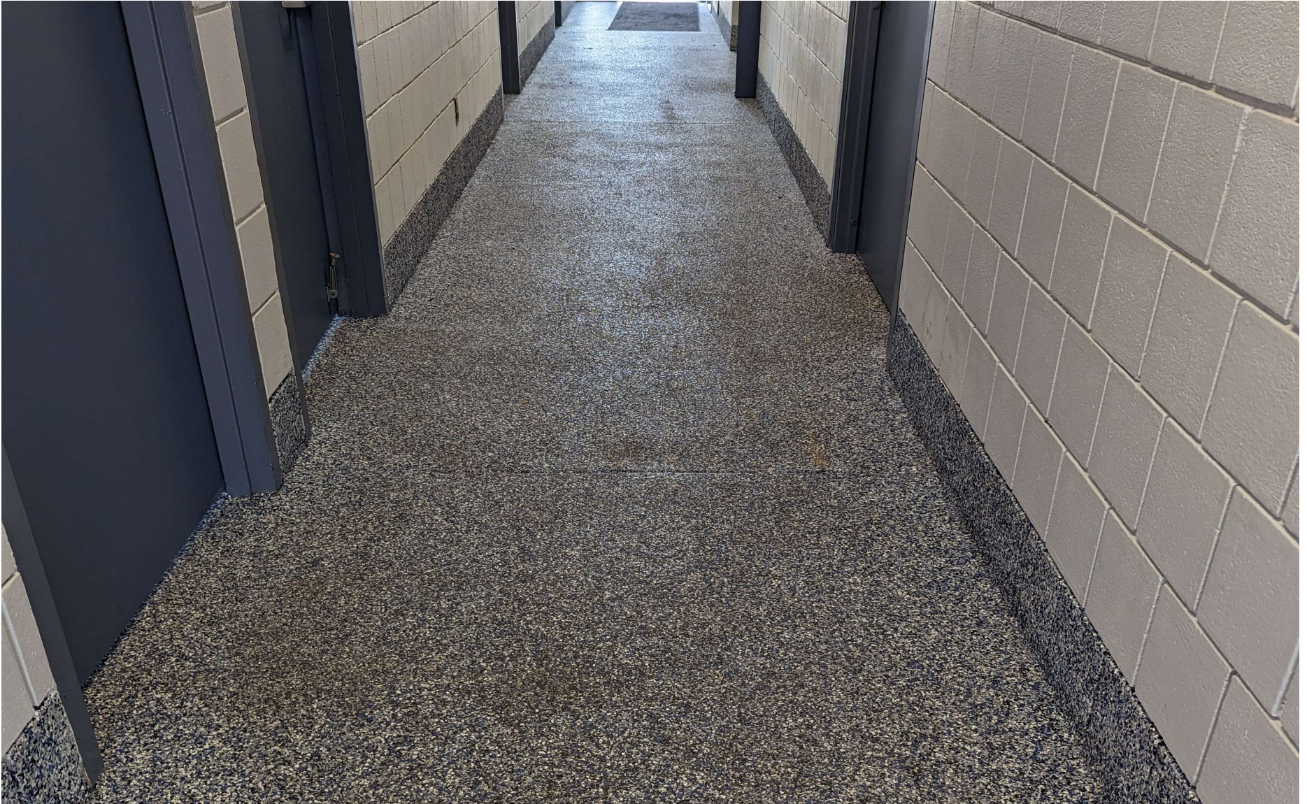
Image #5: FOC Building 1 - Repaired Flooring (AFTER).
