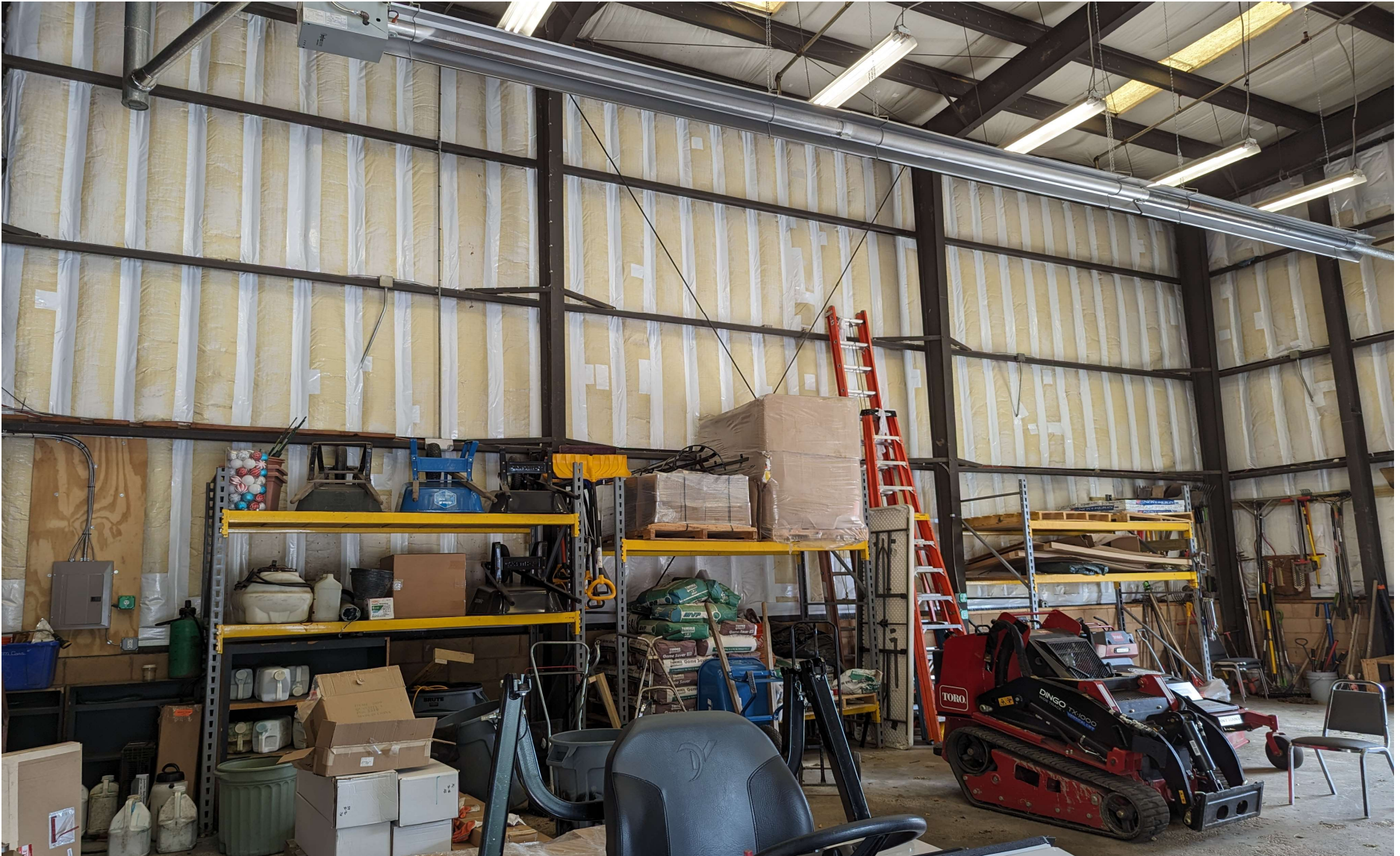
Image #14: FOC Building 4 - Repaired Insulation (AFTER).
