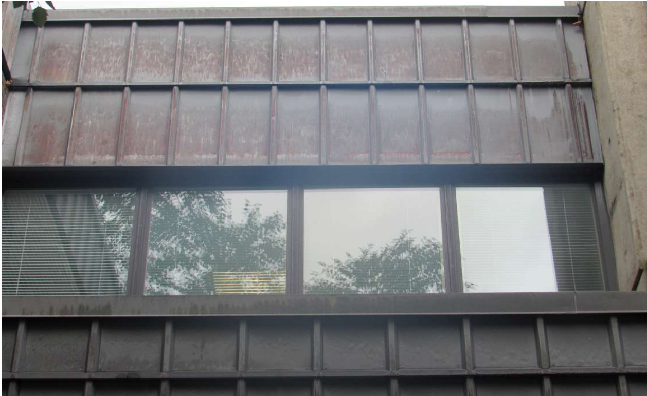
Images #8 and 9: South Main Street Side of City Hall.
