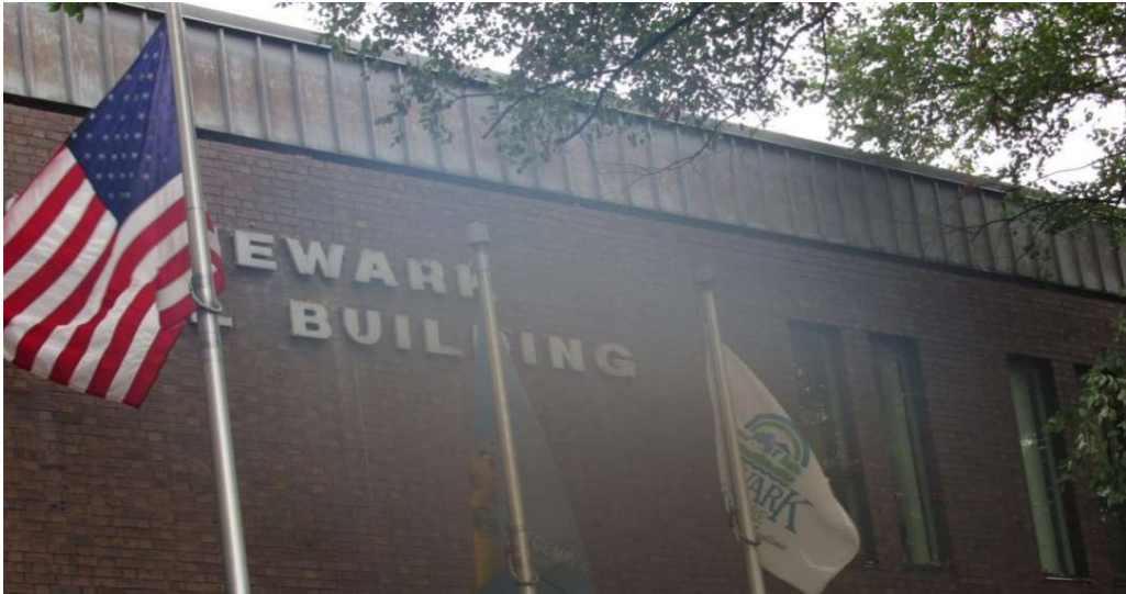
Images #12 and 13: South Main Street Side of City Hall.
