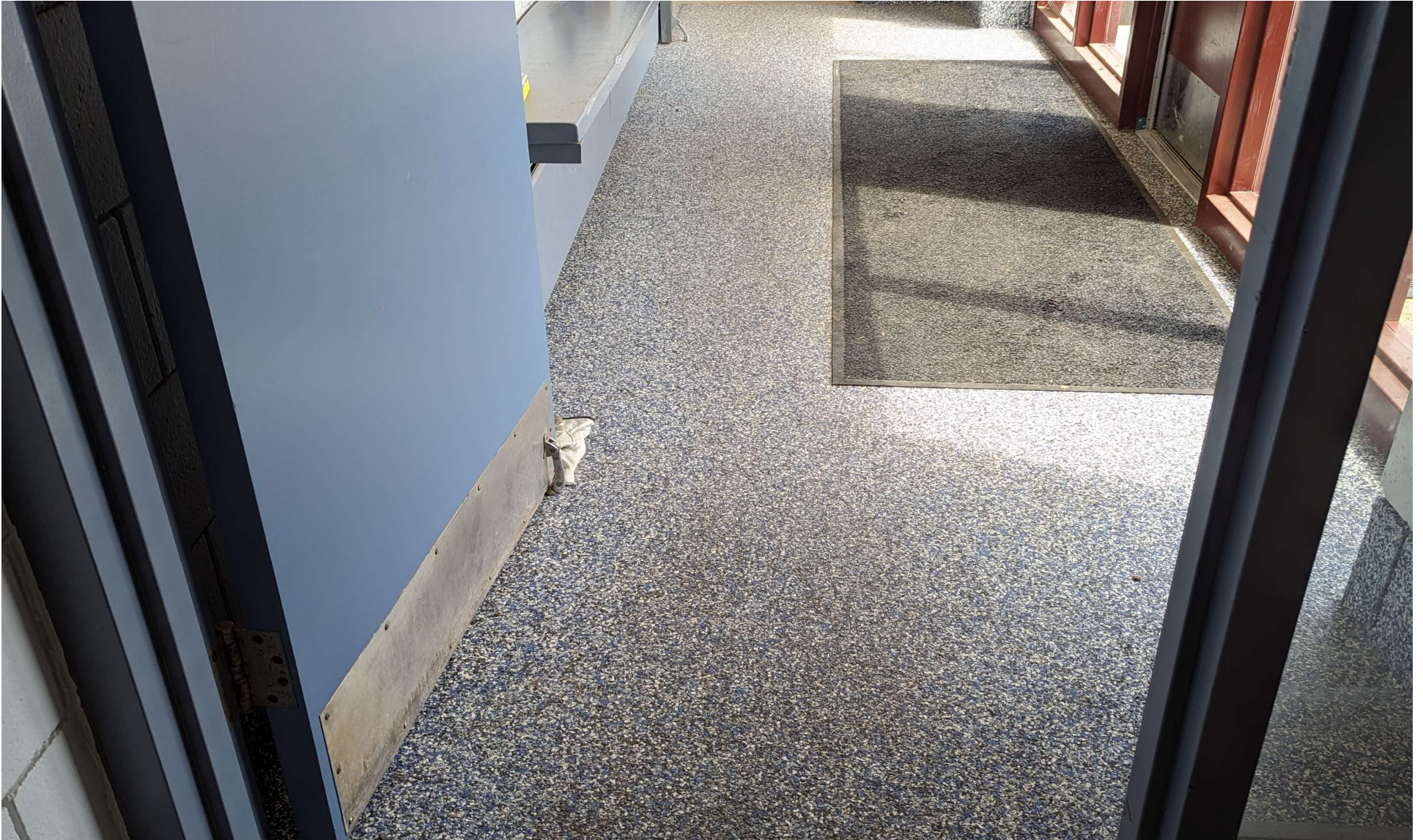
Image #6: FOC Building 1 - Repaired Flooring (AFTER).
