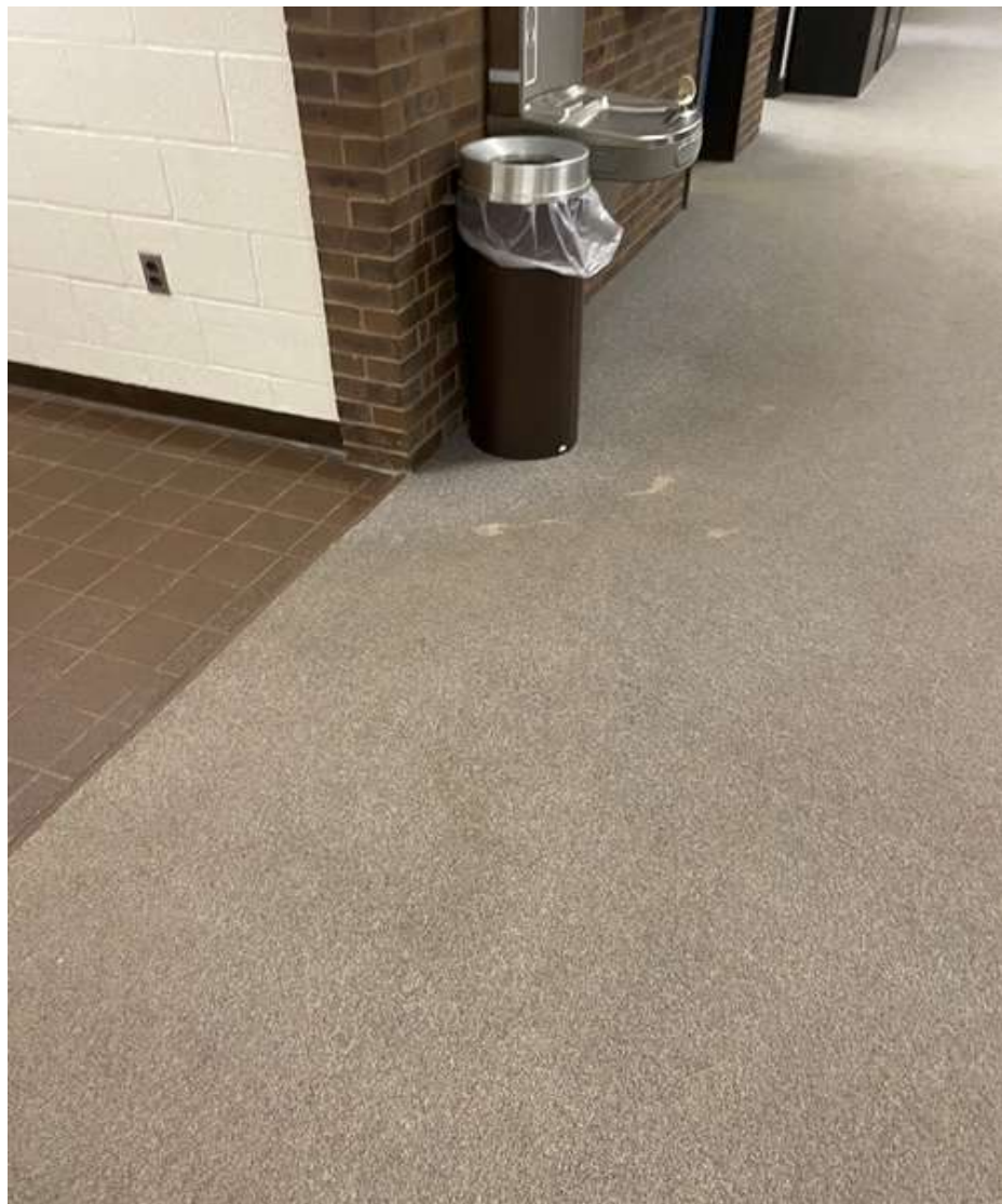
Images #5 and 6: City Hall 2nd floor hallway (BEFORE).
