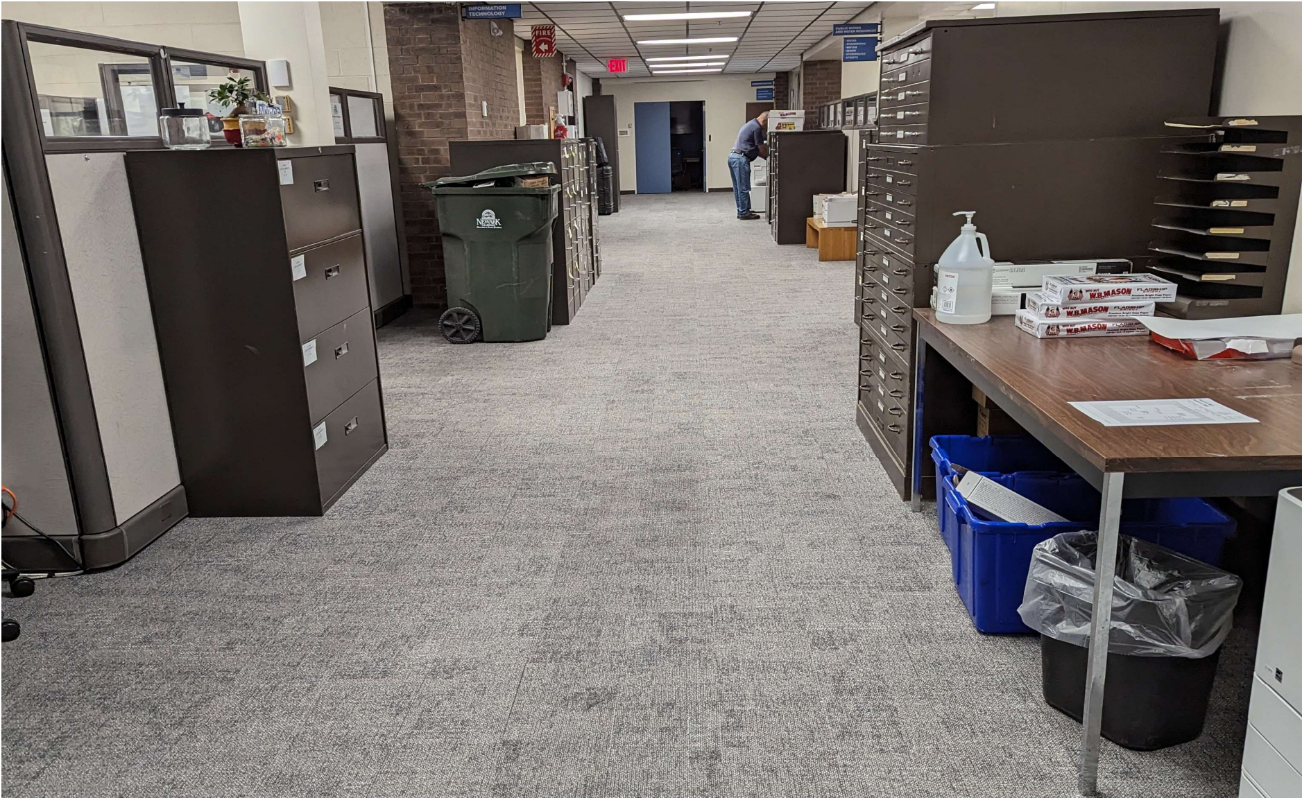
Image #7: City Hall 2nd floor hallway (AFTER).
