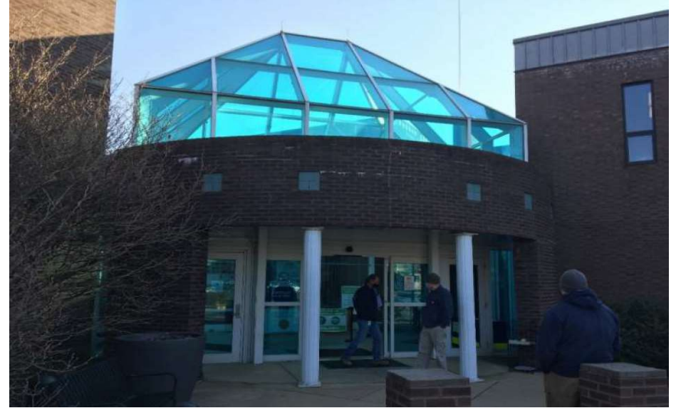
Image #2: Atrium Entrance (BEFORE).
