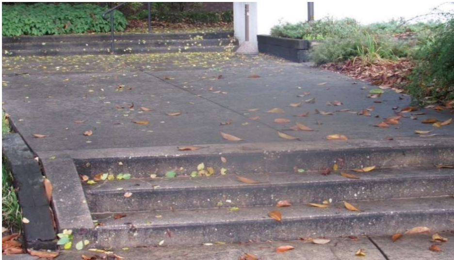
Images #14 and 15: Stairs to City Hall from South Main Street bus station.
