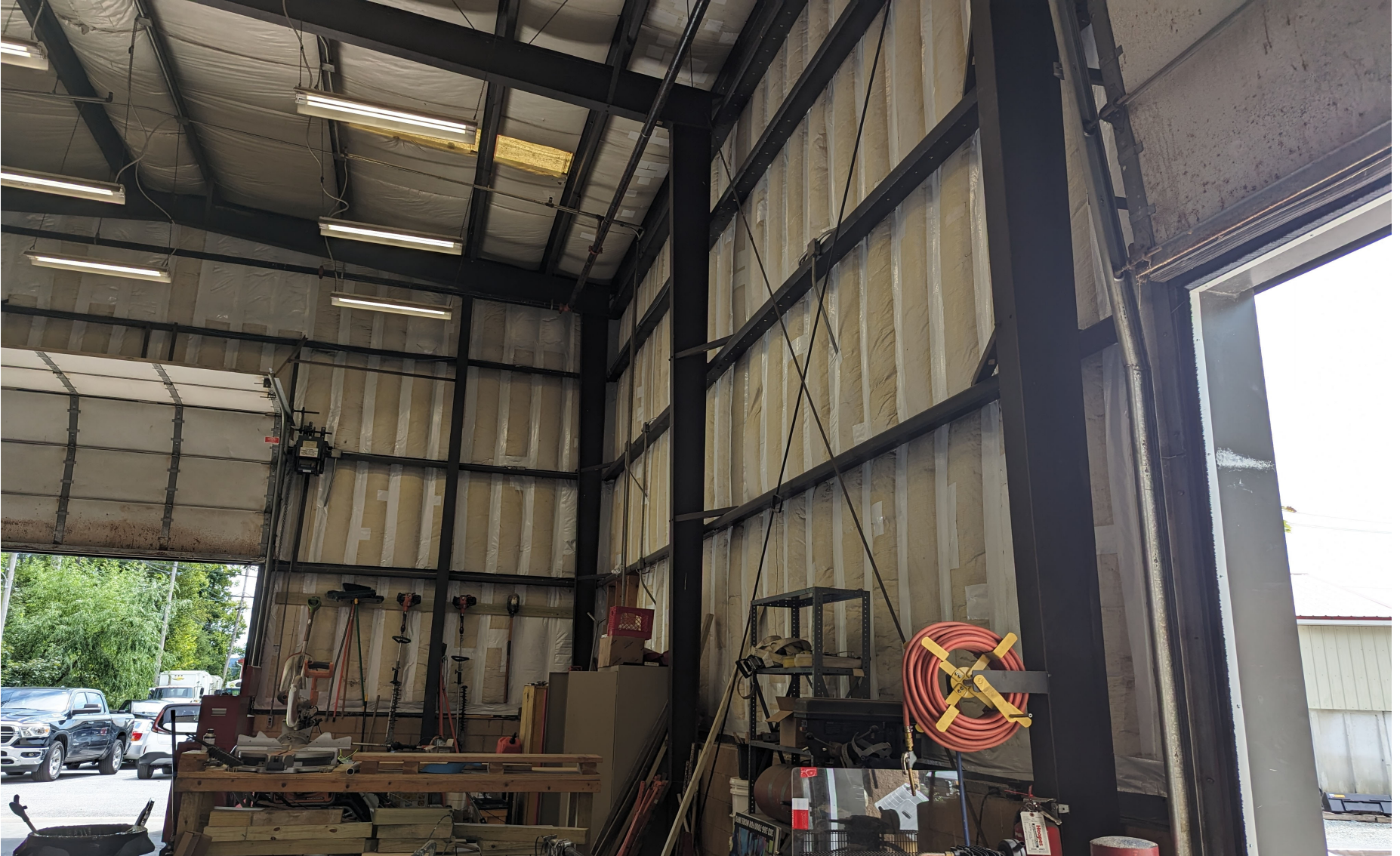
Image #13: FOC Building 4 - Repaired Insulation (AFTER).
