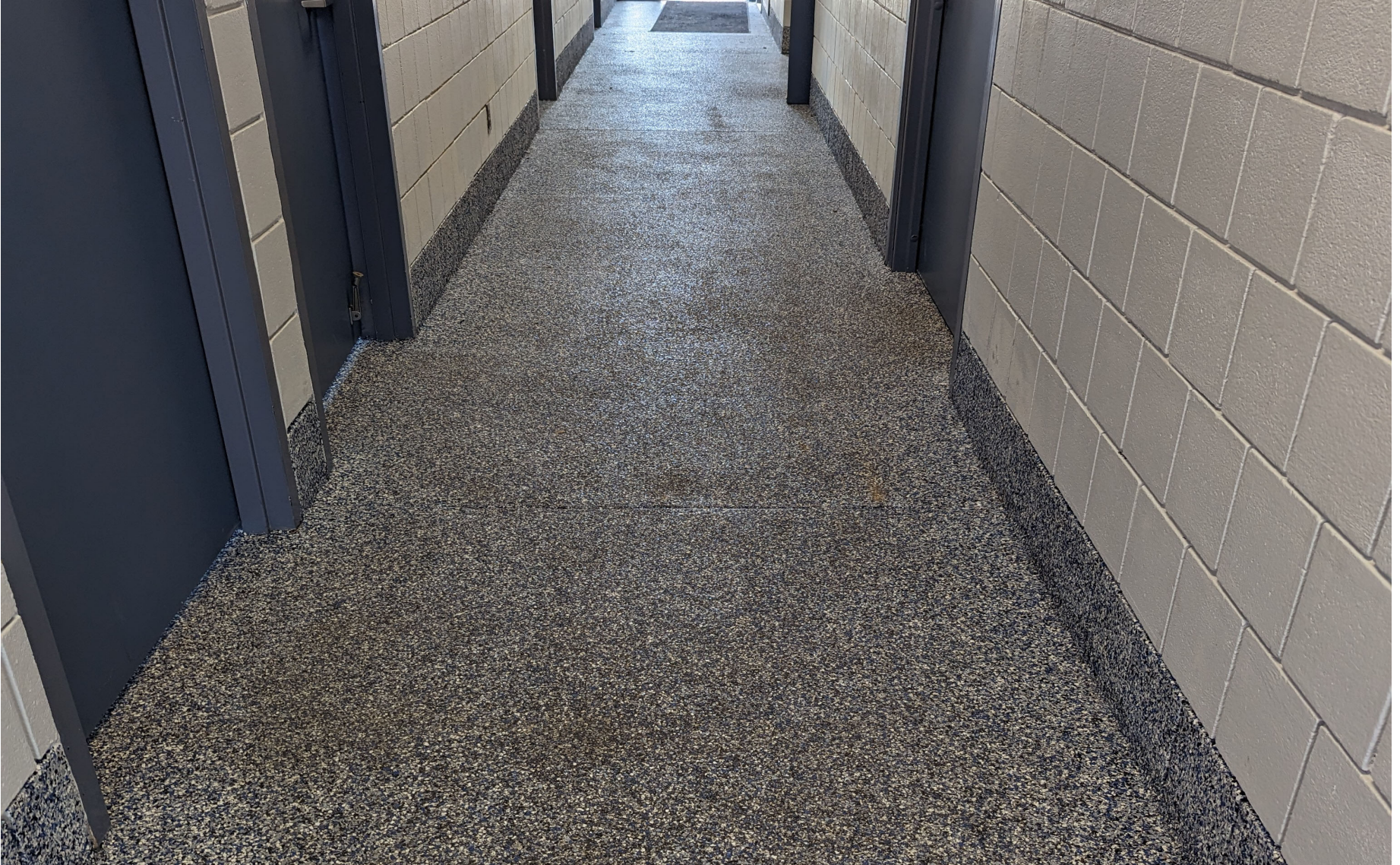
Image #5: FOC Building 1 - Repaired Flooring (AFTER).
