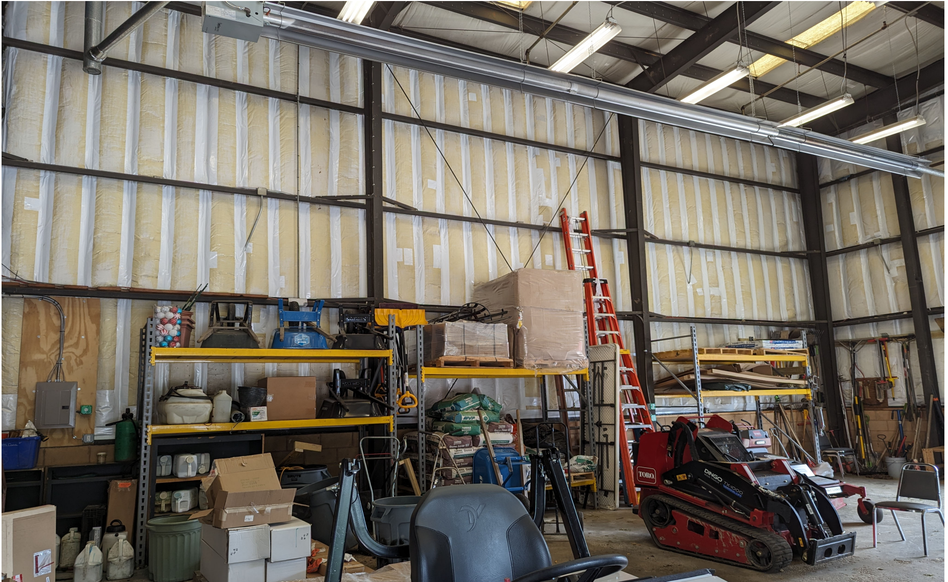
Image #14: FOC Building 4 - Repaired Insulation (AFTER).
