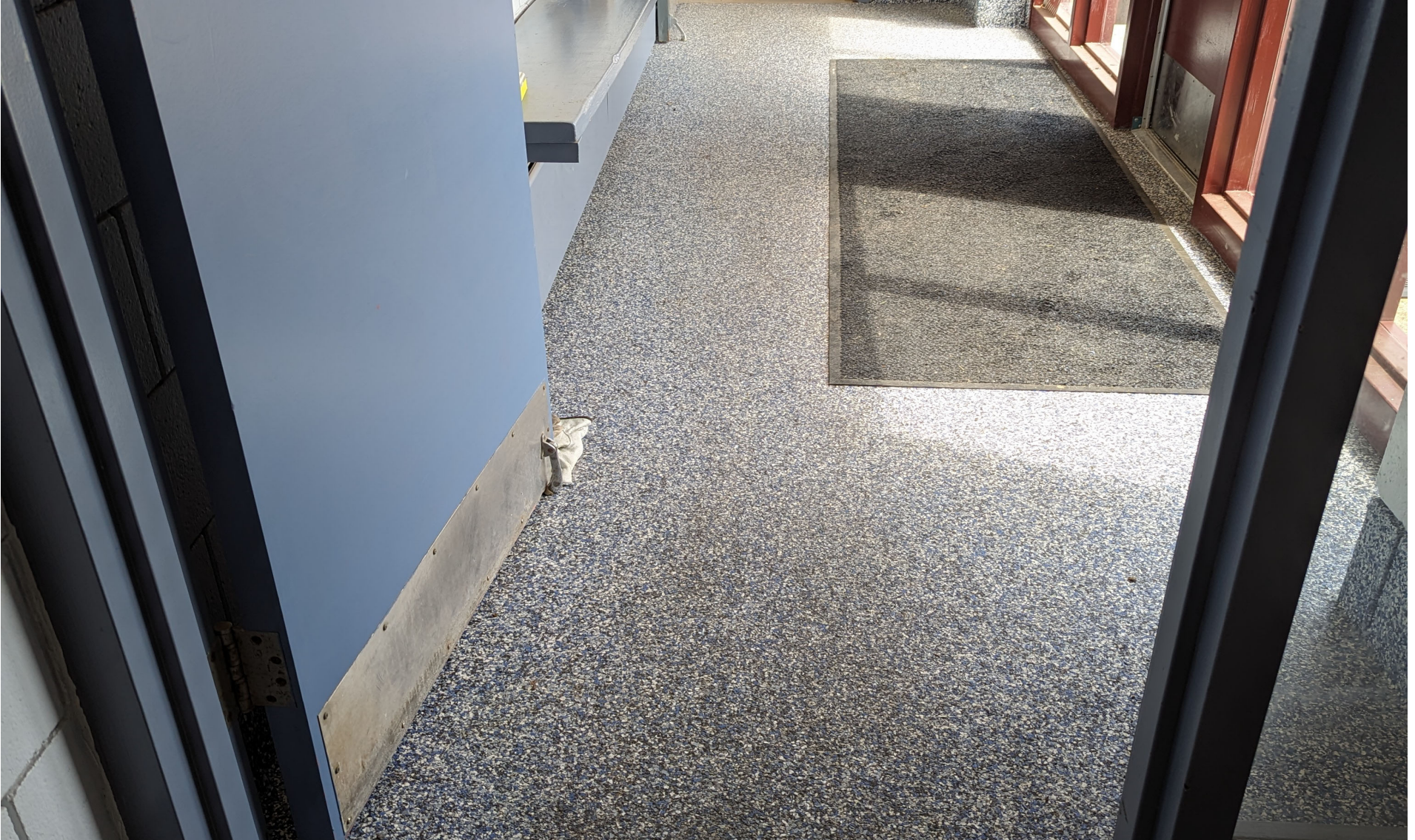
Image #6: FOC Building 1 - Repaired Flooring (AFTER).
