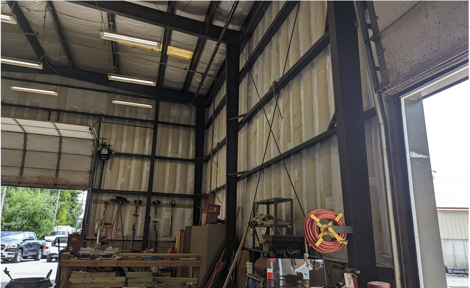
Image #13: FOC Building 4 - Repaired Insulation (AFTER).
