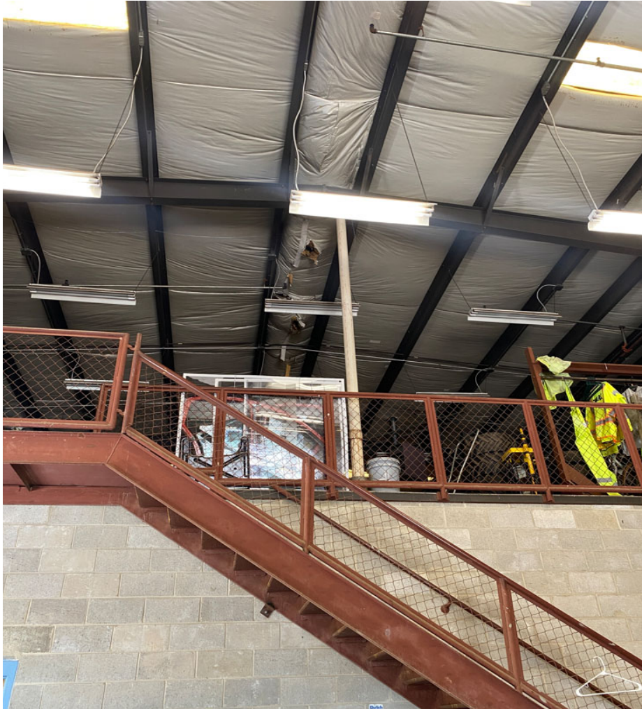
Images #9 and 10: FOC Building 4 [Parks Maintenance break room and offices] (BEFORE).
