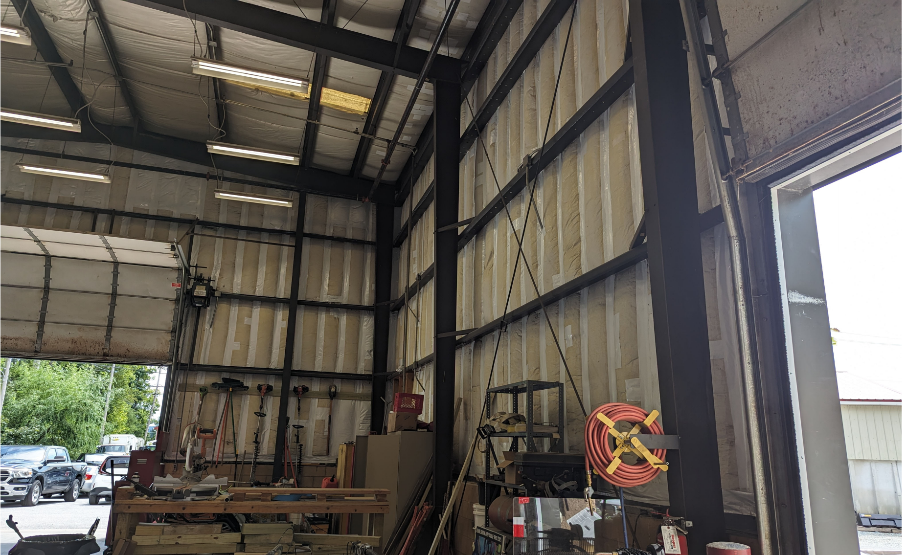
Image #13: FOC Building 4 - Repaired Insulation (AFTER).
