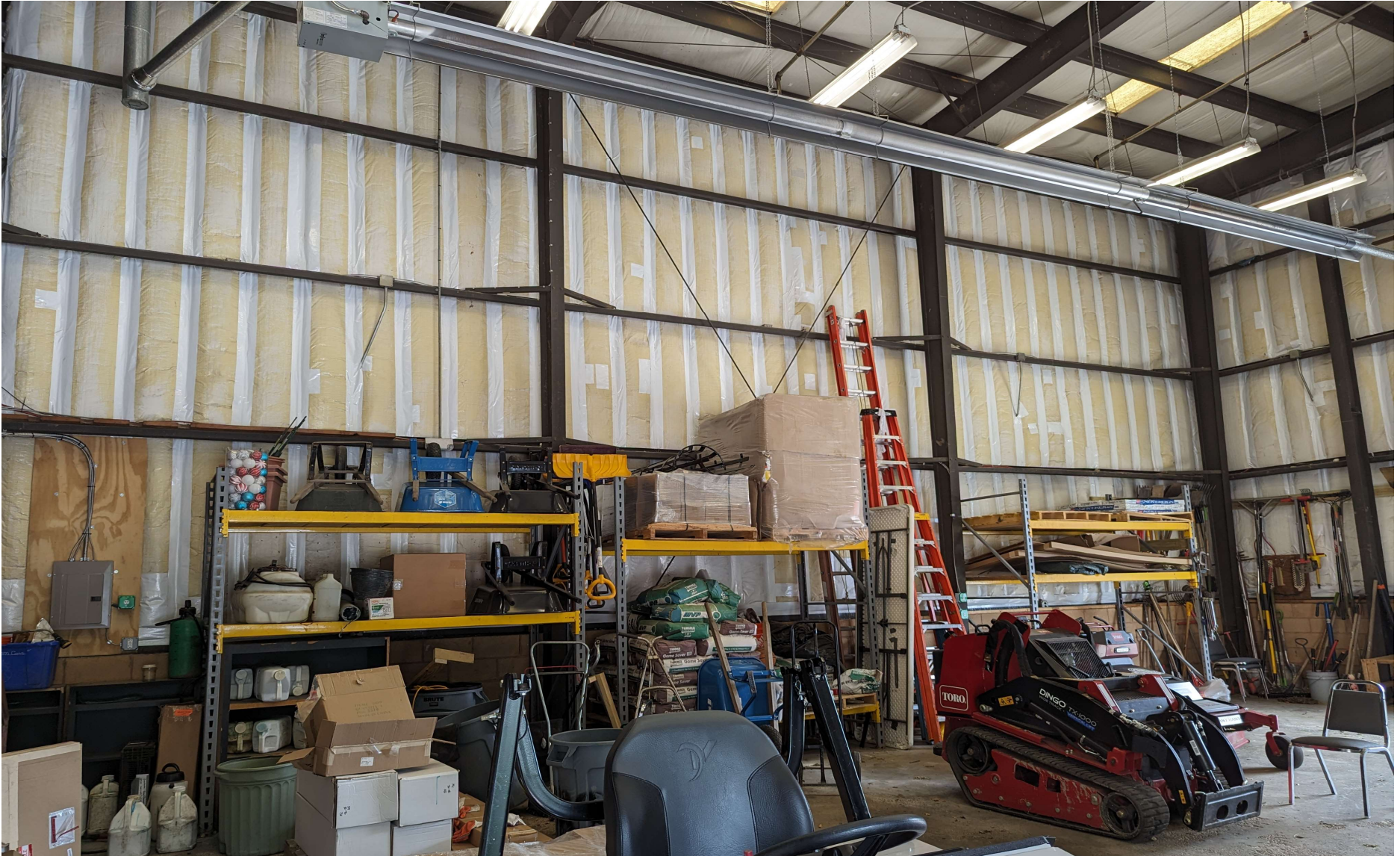
Image #14: FOC Building 4 - Repaired Insulation (AFTER).
