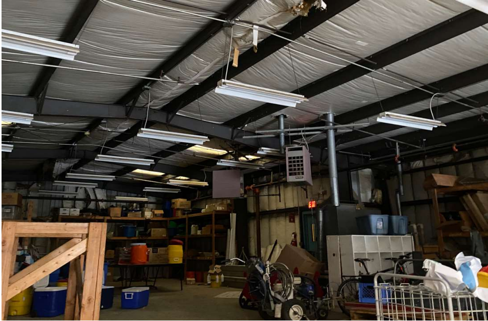
Images #11 and 12: FOC Building 4 [Parks Maintenance break room and offices] (BEFORE).
