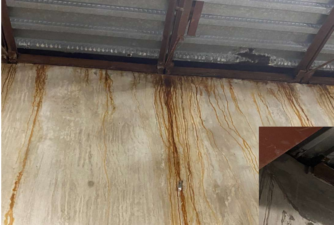
Images #1 & 2: Wall beneath NPD sally port and motorcycle garage
