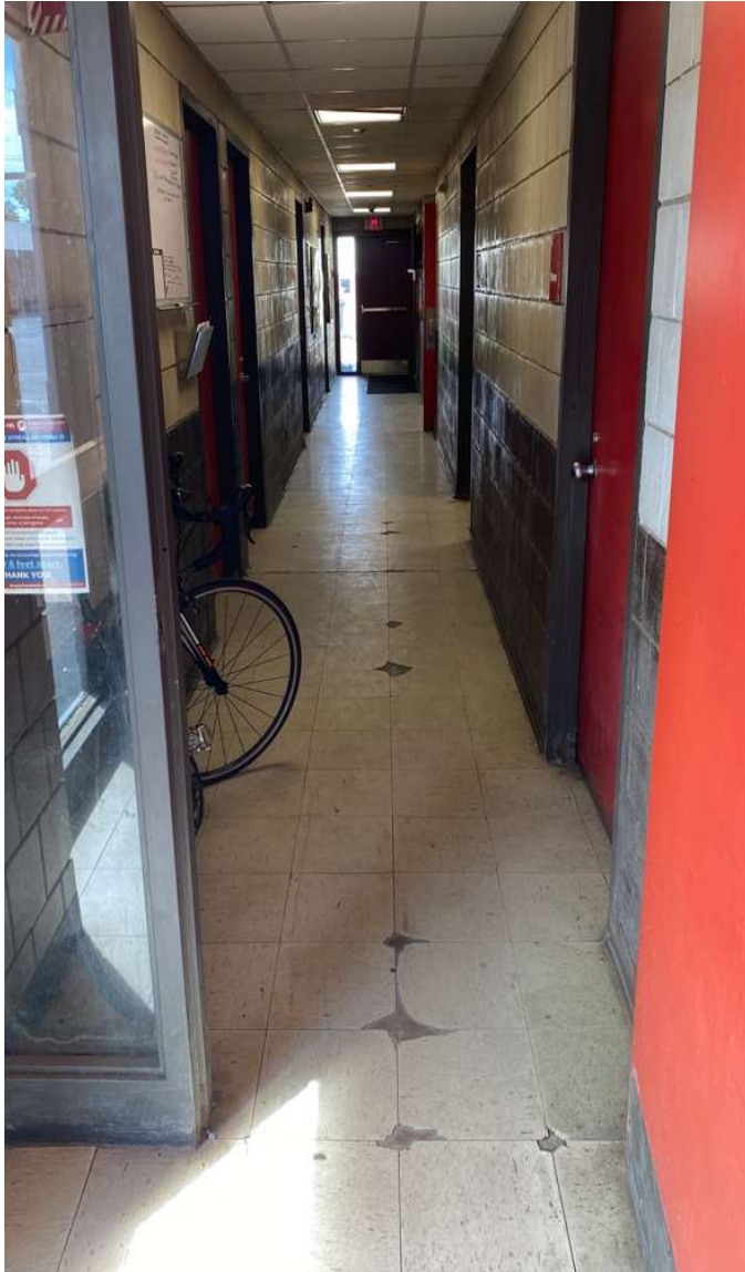
Images #1 and 2: FOC Building 1 [Electric and PWWR offices] (BEFORE).
