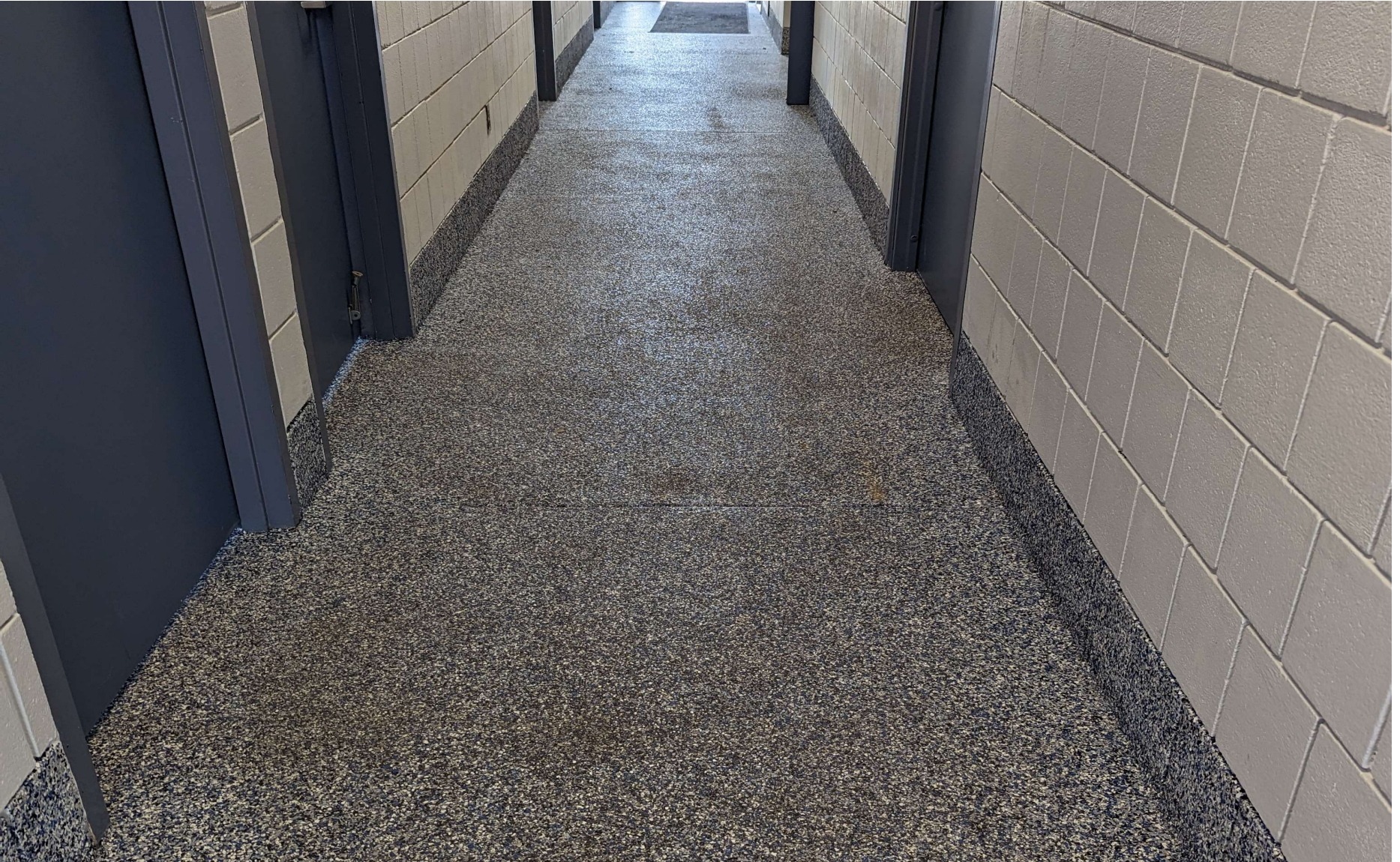
Image #5: FOC Building 1 - Repaired Flooring (AFTER).
