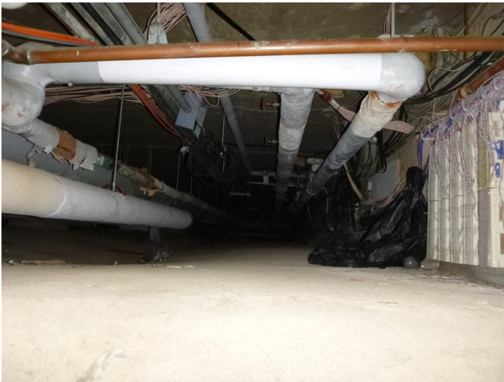
Photograph #5: Crawlspace located in basement of buildings.
