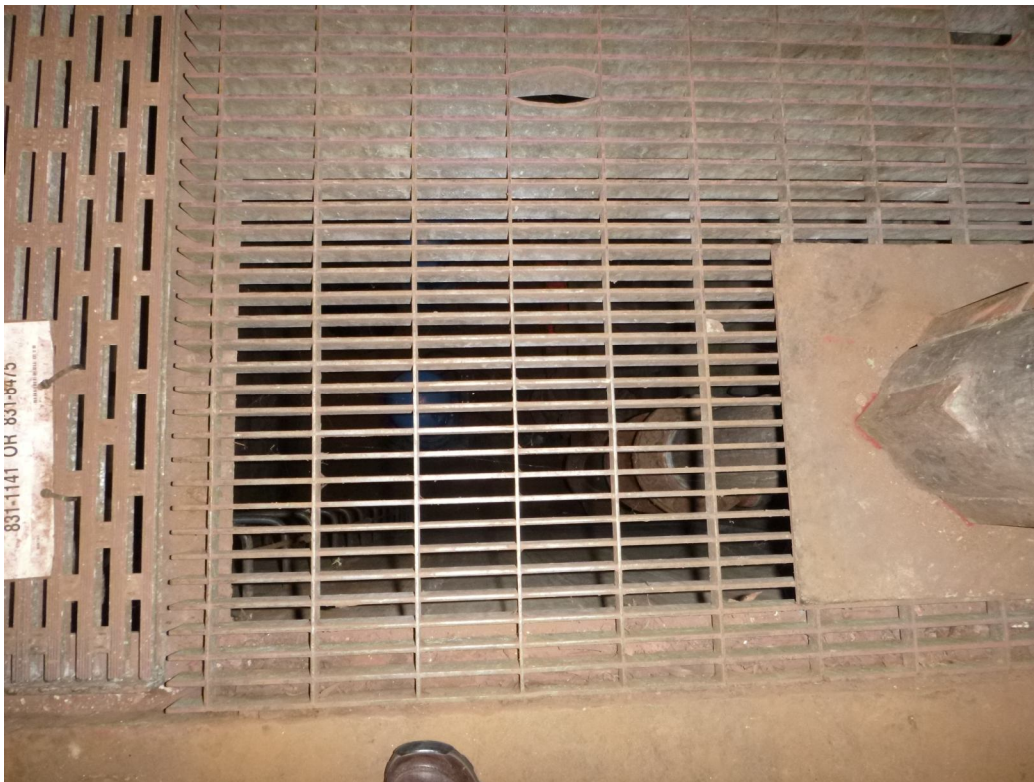
Photograph #3: Sump pit located within Utility Plant.
