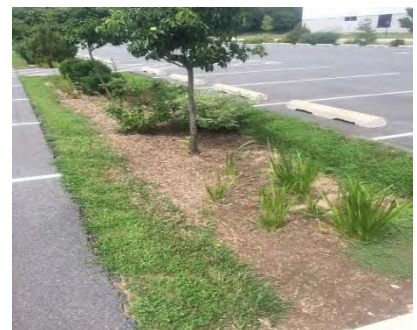
Bioretention Facility or Rain gardens
